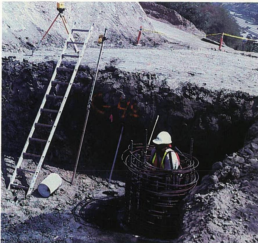
Fig. 16. At some locations, the guideway profile was nearly at ground level. At these locations, the guideway superstructure was supported directly on cast-in-place pile caps.
