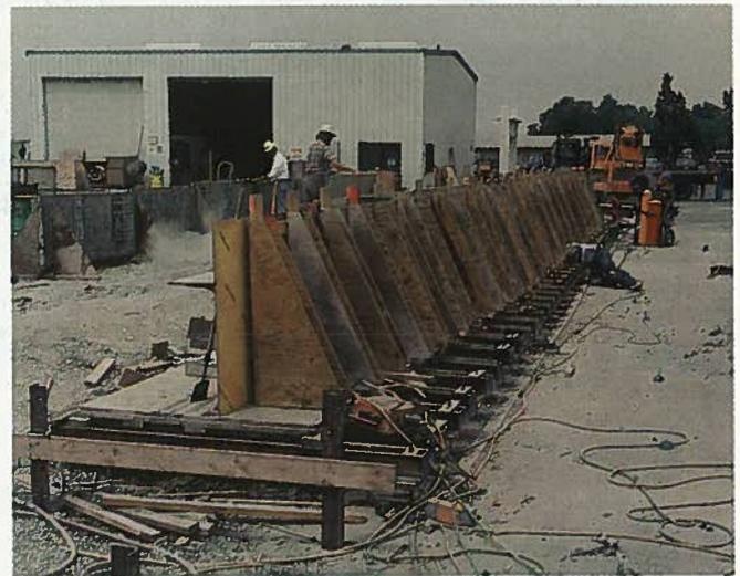
Fig. 26. Web beam forms were made from plywood secured to a series of 90-degree timber frames. Side forms were flat planks sheathed with plywood, thus creating a flexible yet not too rigid form.
