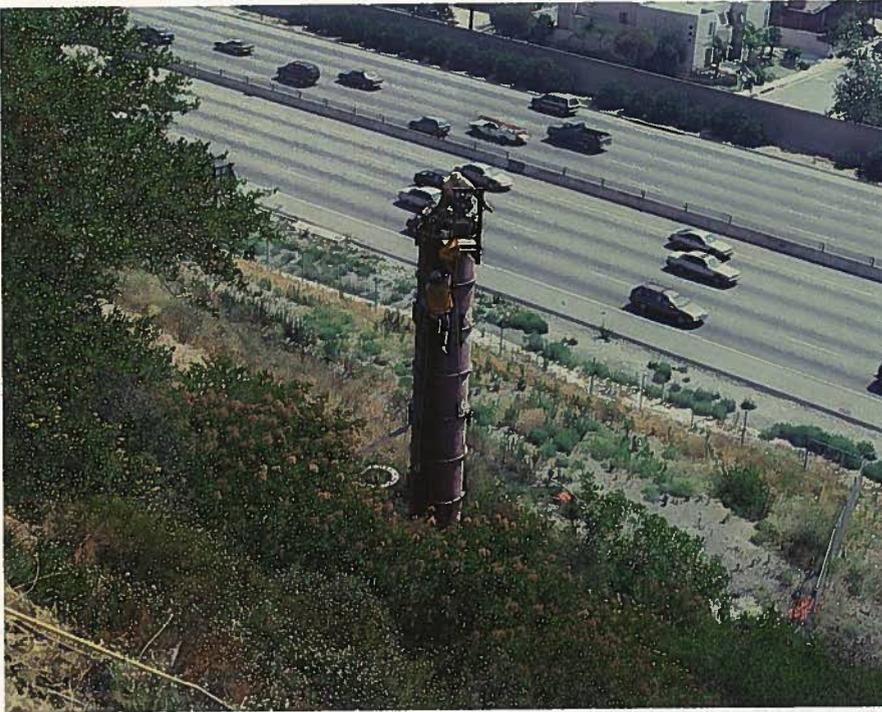
Fig. 13. Some column locations were only accessible by foot.
