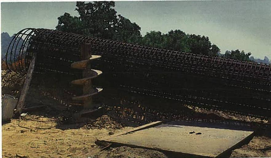
Fig. 14. Reinforcing steel cages for drilled shaft foundations and columns were over 30 m (100 ft) long.
