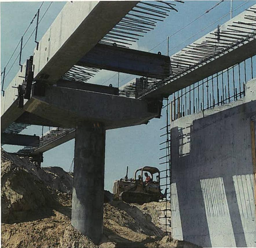
Fig. 19. W30 steel sections were used to tie the web beams securely together after erection.
