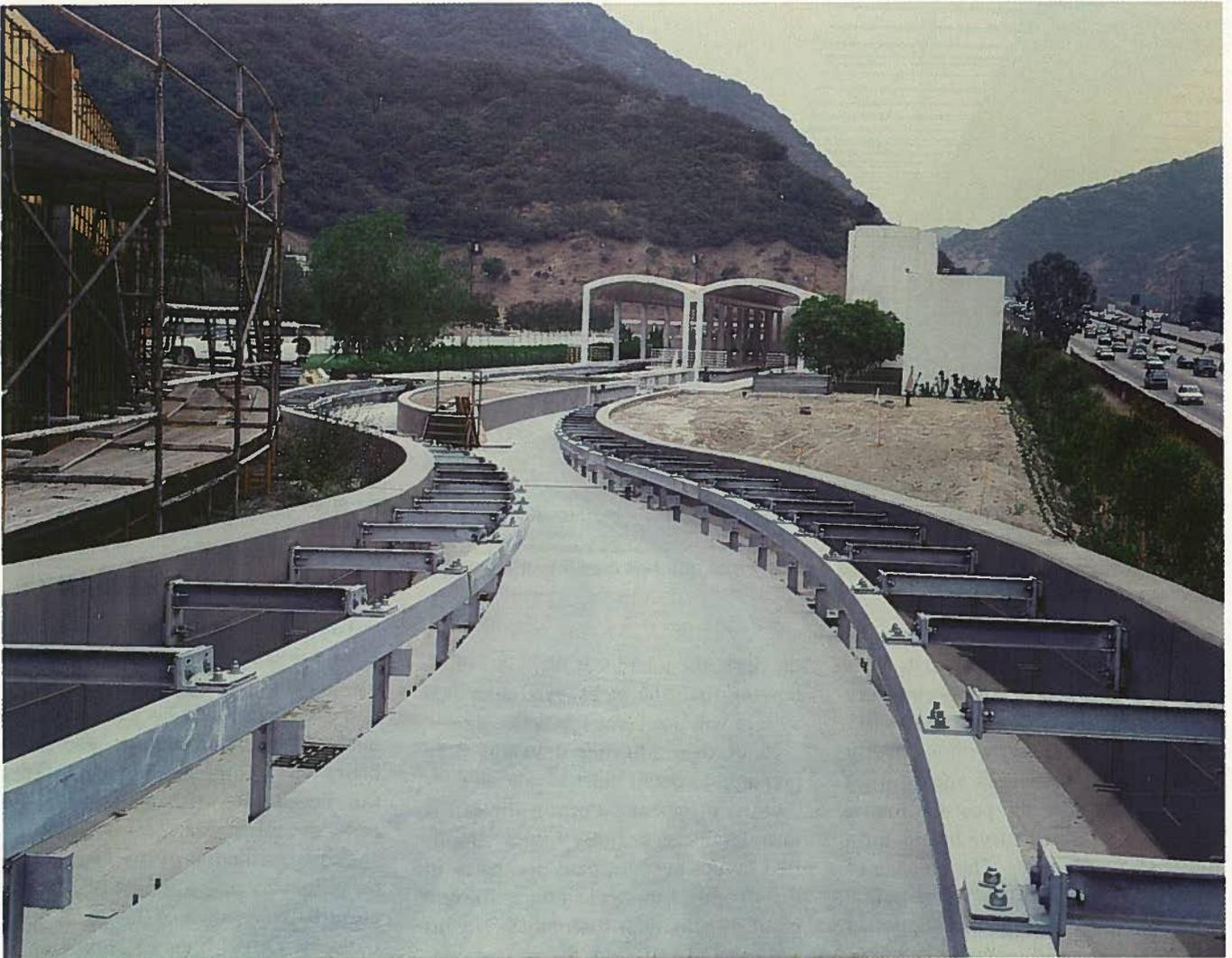
Fig. 24. The flying surface and steel guide rails are ready to receive the rope sheaves and power rails.
