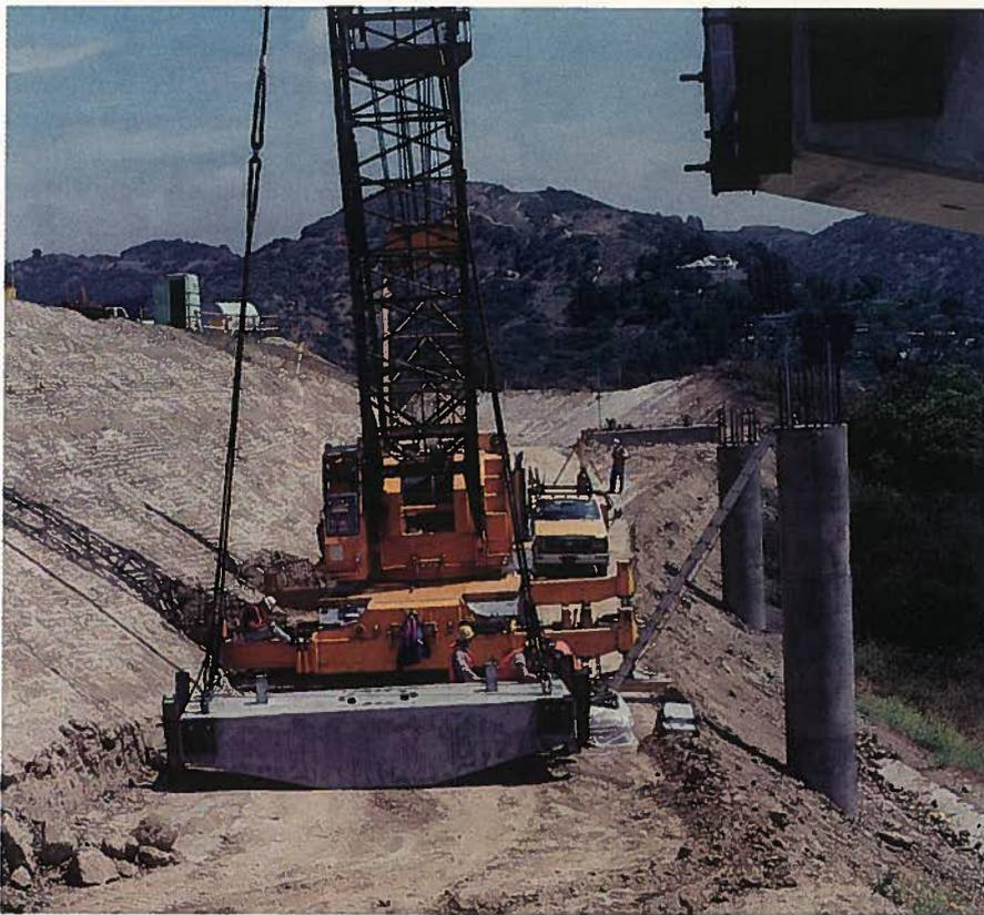
Fig. 11. The erection crane was able to back out a narrower access road without cross-heads atop the columns. A precast concrete cross-head is being rigged for erection.
