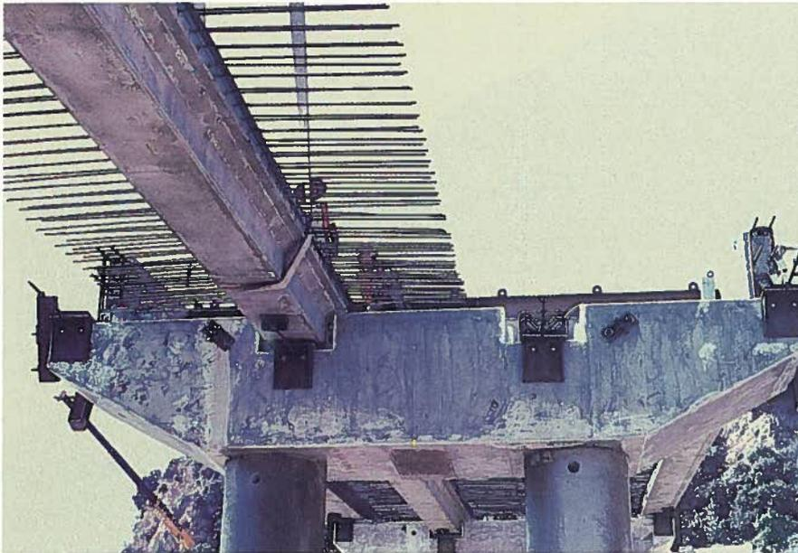
Fig. 21. Stem beams in the bypass area were set into notches cast into the precast concrete cross-heads.
