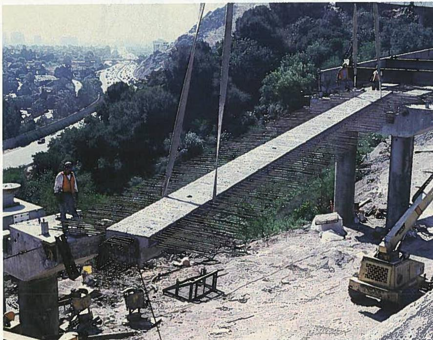
Fig. 20. In the bypass area, stem beams were used to stiffen the section.
