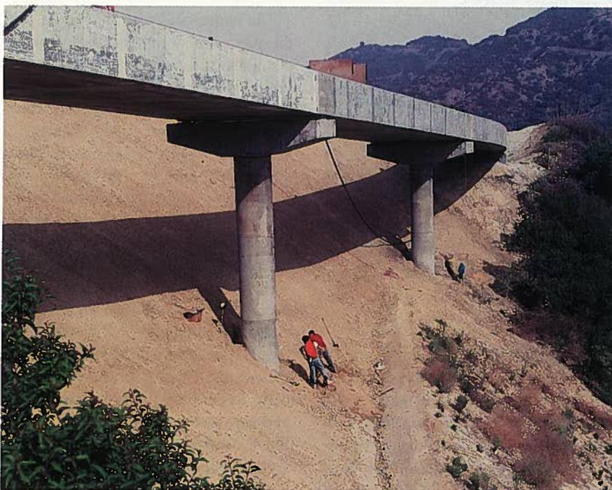
Fig. 12. Guideway columns are located on steep hillsides.
