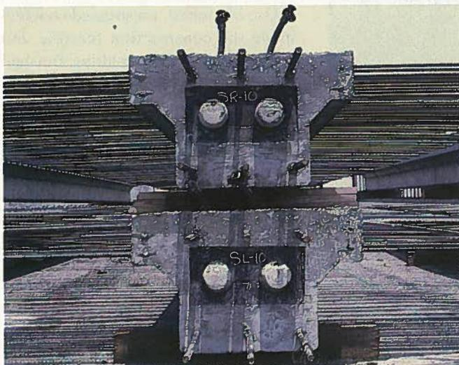
Fig. 25. Two stem beams in the storage yard are ready for transport to the site. Precast concrete beams were post-tensioned in the yard to carry their own weight and construction loads.
