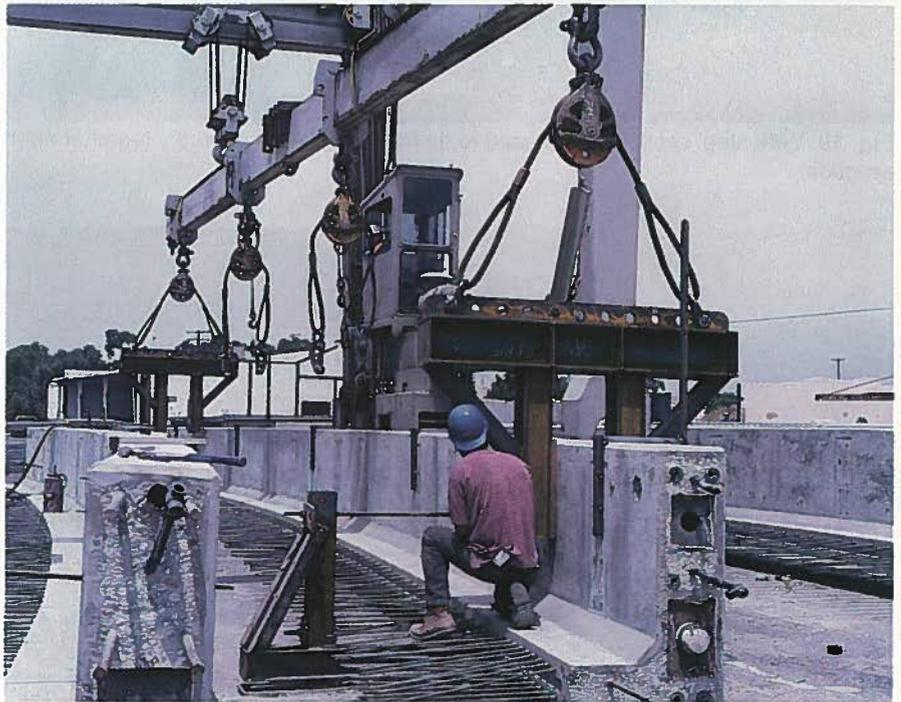
Fig. 18. Special lifting frames were fabricated to allow picking outside the center of the web beam cross section.
