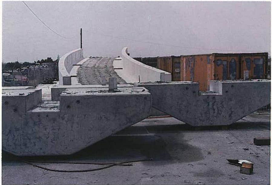
Fig. 17. Prior to production, a full-scale mock-up was constructed at the precast manufacturing yard.
