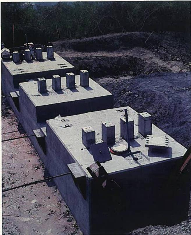
Fig. 9. Multiple steel lugs and bearings were required to transfer earthquake shear forces from the guideway superstructure to this pier.
