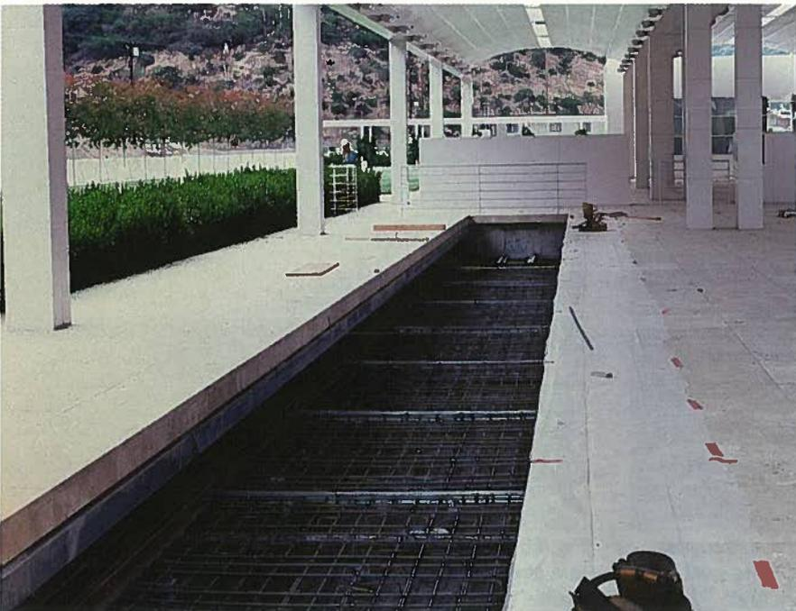
Fig. 23. Reinforcing steel placed in the flying surface at the Entry Station.
