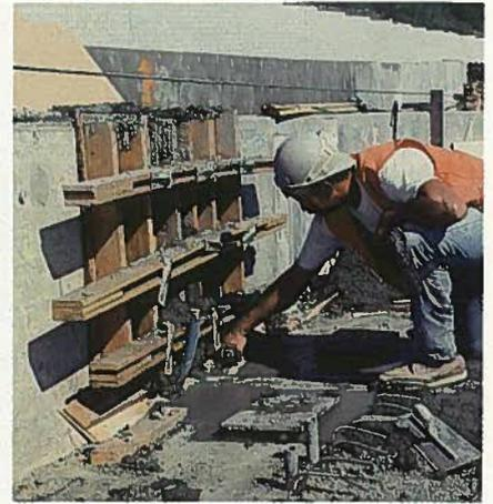
Fig. 22. After precast concrete beams were erected, closure pours were cast to make the precast units into four- to six-span continuous beam units.
