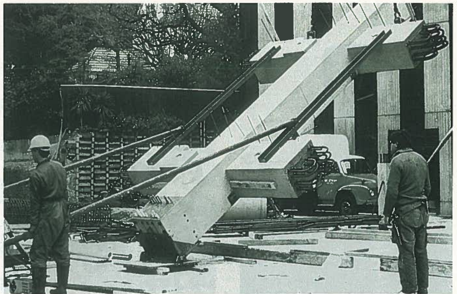
(a) Double cruciform-shaped precast concrete frame unit being lifted (Ref. 16)
