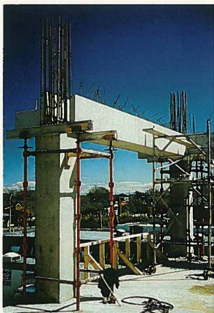
Fig. 16. Construction of a moment resisting frame using precast concrete U-beams.
