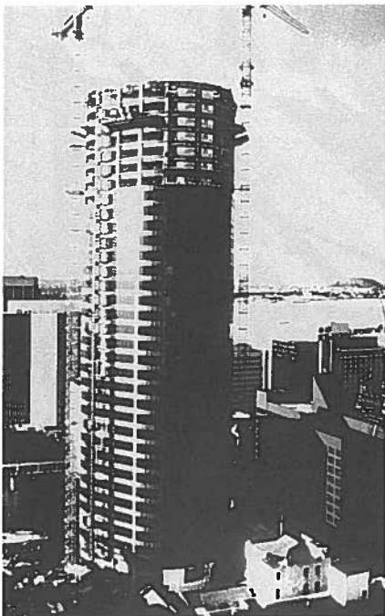
(a) Construction overview of building
