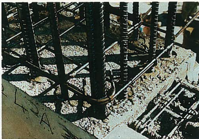
Fig. 7. Construction of a 22-story building using System 2 in New Zealand.
