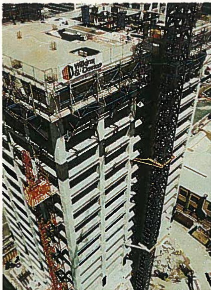
(a) Structure of reinforced concrete perimeter frame
