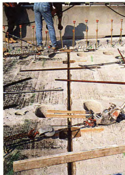
Fig. 2. Transverse joint between precast panels during construction.
