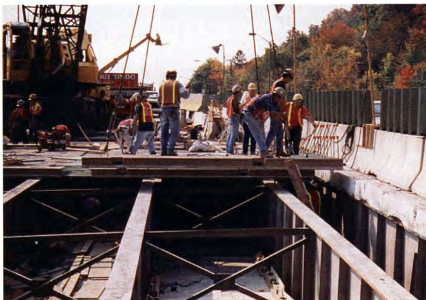
Fig. 1. View of system under construction.
