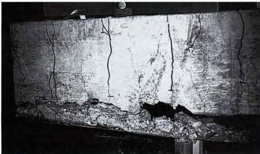
Fig. 3(e). Beam at failure.
