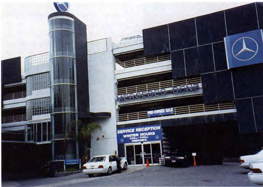
Fig. 12. Auto Steigler Parking, Encino. Only minor cracking occurred (Garage 28).
