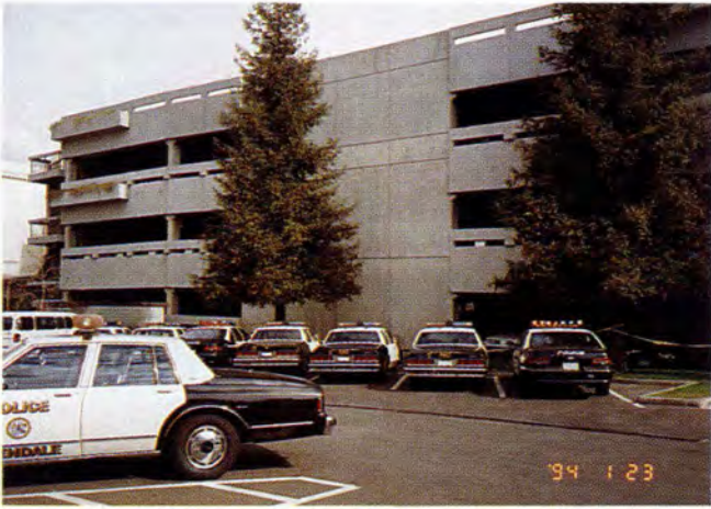
Fig. 17. Glendale Civic Center Parking. Undamaged west face (Garage 7).
