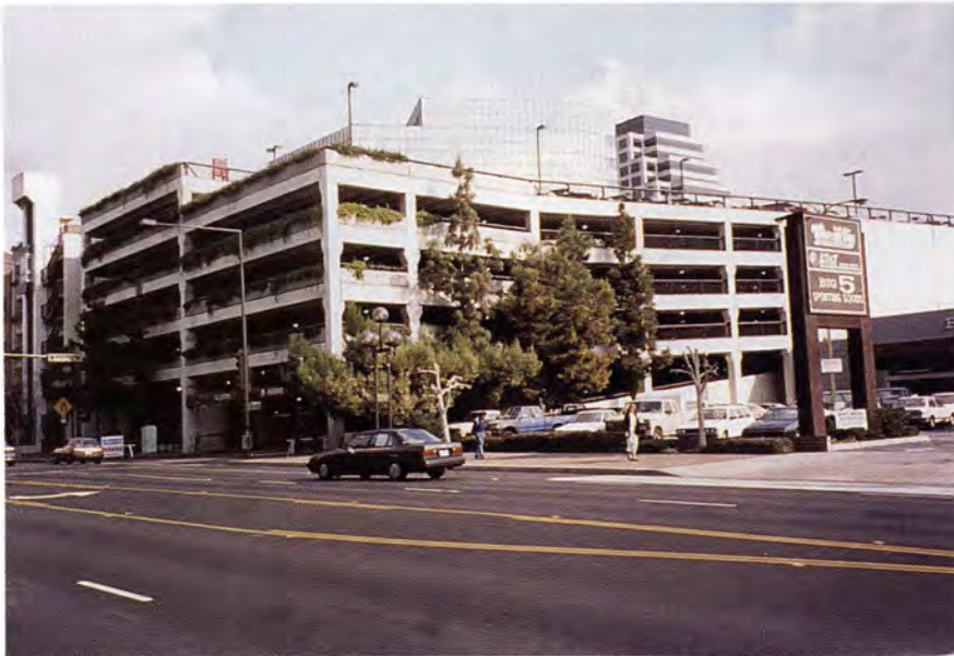
Fig. 22. Glendale Galleria, Central Avenue Parking. Note undamaged garage (Garage 25).
