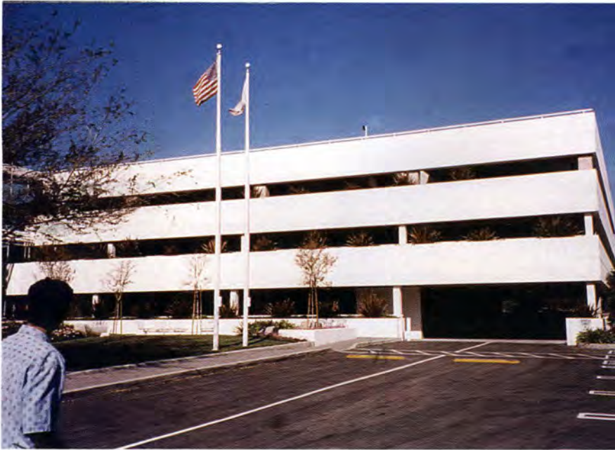
Fig. 10. Undamaged Litton Industries garage, Chatsworth, about 1 mile (1.6 km) east of epicenter (Garage 20).
