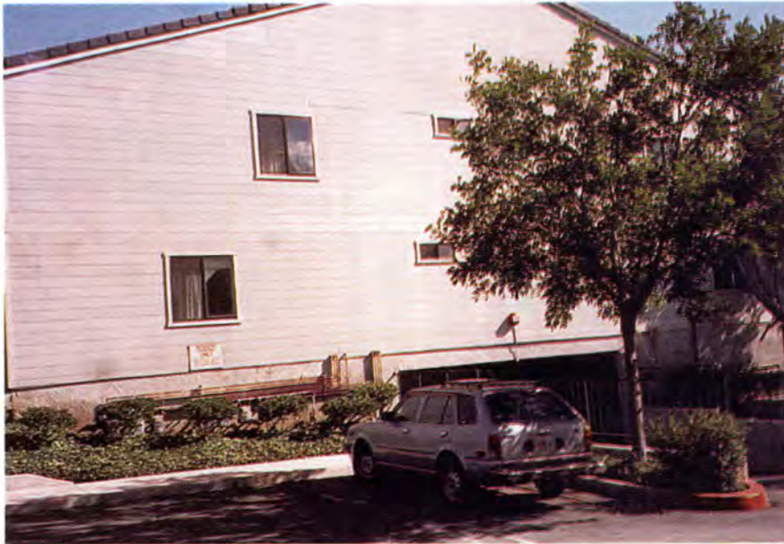
Fig. 34. Wood frame of Devonshire Apartments, Northridge.
