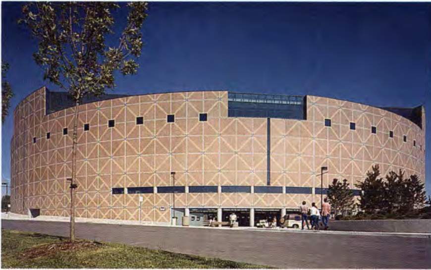
Fig. 7a. The Palace of Auburn Hills, Auburn Hills, Michigan, is clad with 9 in. (225 mm) thick curved precast concrete panels cast with a contrasting basketweave pattern of 8 in. (200 mm) square, 2 in. (50 mm) thick brick units and a rectilinear grid of blue-green glazed brick. Architect: Rossetti Associates, Detroit, Michigan.
