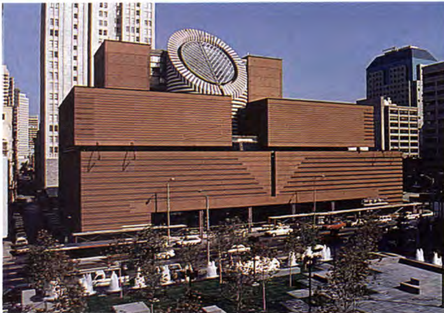
Fig. 5a. The patterned facade on the San Francisco Museum of Modern Art has 1 in. (25 mm) thick brick on 9 in. (225 mm) thick precast concrete panels. Most panels measure 10 x 28½ ft (3 x 8.7 m) and contain 1500 to 2300 bricks per panel. Project Architect: Mario Botta, Lugano, Switzerland. Architect of Record: Hellmuth, Obata and Kassabaum, San Francisco, California.
