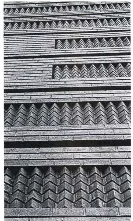
Fig 5b. Closeup view of patterned facade.
