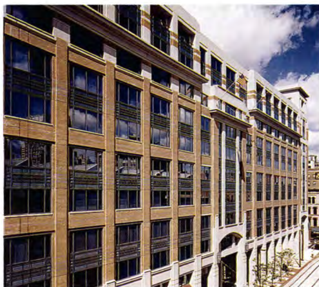
Fig. 26. The column covers on the City Crescent Federal Office Building, Baltimore, Maryland, have field-laid bricks that are supported on shelf angles welded to the precast concrete. Architect: The Weihe Partnership, Washington, D.C.
