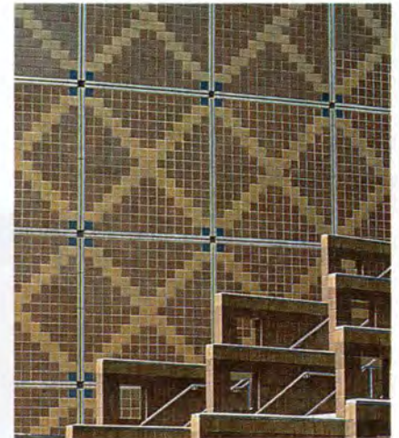
Fig. 7b. Each panel is 20 ft (6 m) wide by 10 ft (3 m) high with a false joint in the middle. The intersection of the grids is accentuated by a cluster of glazed tile units. The panel edges are exposed concrete and deeply chamfered to provide shadow lines.
