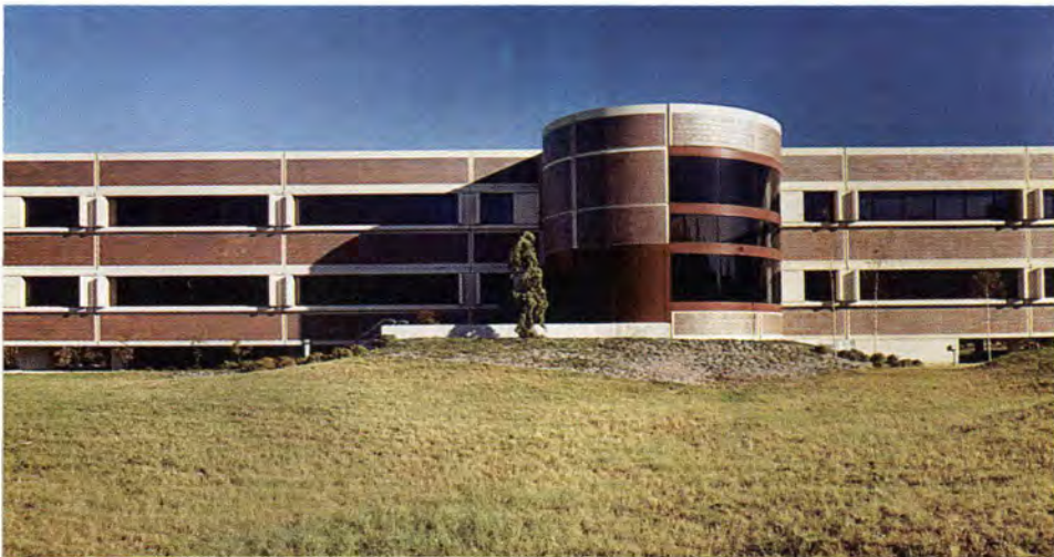
Figs. 9a and 9b. Spandrels and wall panels on Sylvan Corporate Center, Englewood Cliffs, New Jersey, have integrally cast 8 in. (200 mm) square brick-colored tiles with pigmented mortar. A beige band of concrete surrounds the tile field. Architect: Herbert Beckhard Frank Richlan & Associates, New York, New York.
