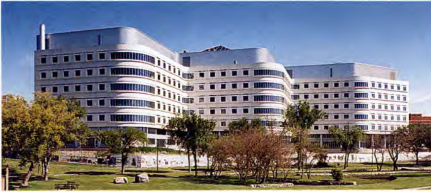
Fig. 21a. Saskatoon City Hospital walls are precast concrete sandwich panels incorporating insulation and a rain screen, with ceramic tile on the exterior. Architect: City Hospital Architects Group, Inc., Saskatoon, Saskatchewan, Canada, a Joint Venture of Folstad & Friggstad Architects, Billington Poon Associates Ltd. and Arthur Erickson Architects.
