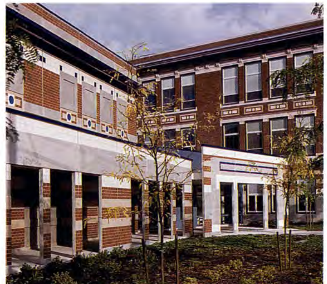
Fig. 22. The Ravenna Eckstein Community Center in Seattle, Washington uses precast concrete panels articulated with reveals and recesses varying from \frac{3}{4} to 1\frac{1}{2} in. (19 to 35 mm) to reflect the adjacent 1911 school's proportions. Ceramic tile was then selectively field-laid on the concrete to reference the school's brick and terra cotta banding and details. Architect: ARC Architects, Seattle, Washington.
