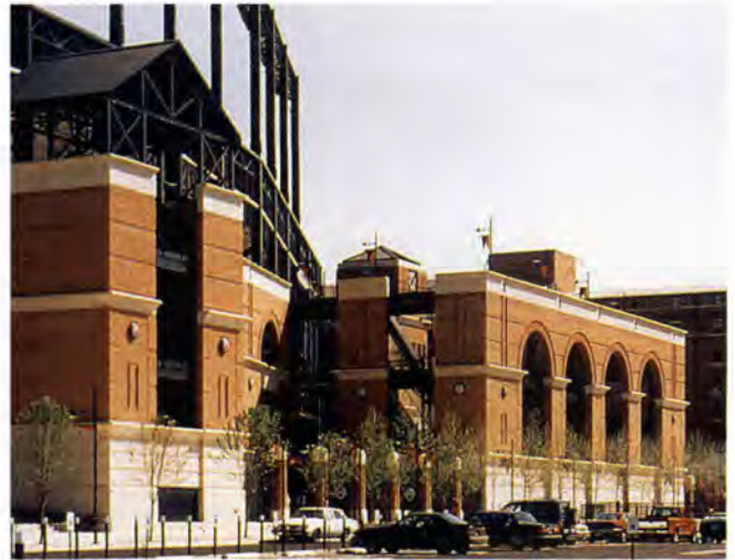
Fig. 24. The low-scaled, arched facade of Oriole Park at Camden Yards presents itself in the form of elaborate cornices and rustication joints. Brick anchored to dovetail slots in the precast concrete was field-laid on concrete ledges via scaffolding following precast concrete erection. Architect: Hellmuth, Obata and Kassabaum Sports Facilities Group, Kansas City, Missouri.
