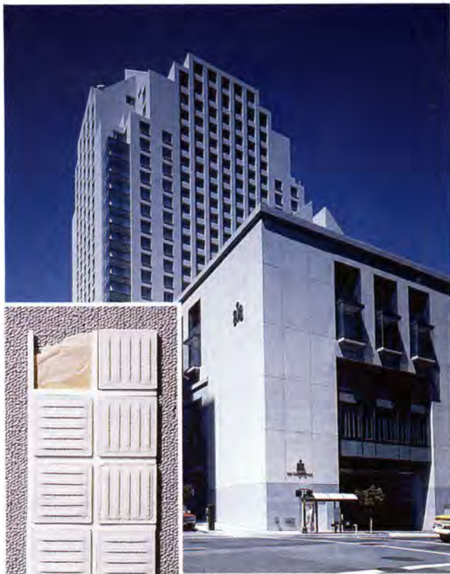
Figs. 15a and 15b. The Nikko Hotel, San Francisco, California uses 2 x 2 in. (50 x 50 mm) tiles, which were supplied face-mounted on 12 in. (300 mm) square paper sheets (see inset). Architect: Whisler-Patri, San Francisco, California.
