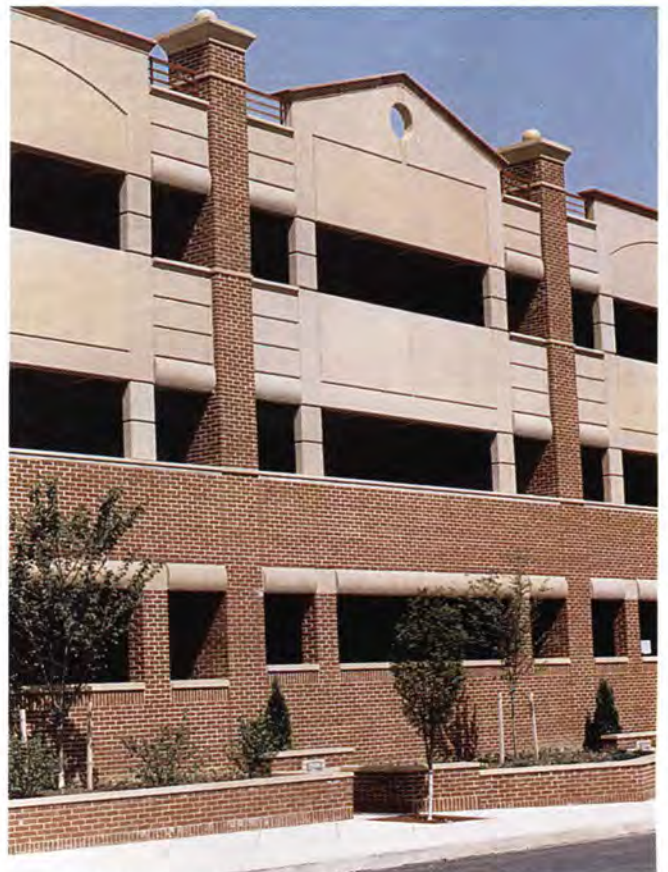
Fig. 19. Spandrels on the Poplar and Walnut Parking Garage, Reading, Pennsylvania, are designed with segmented bullnose ledges and integral copings. The ledges support field-laid brick. Architect: Synergetics Architects, Reading, Pennsylvania.
