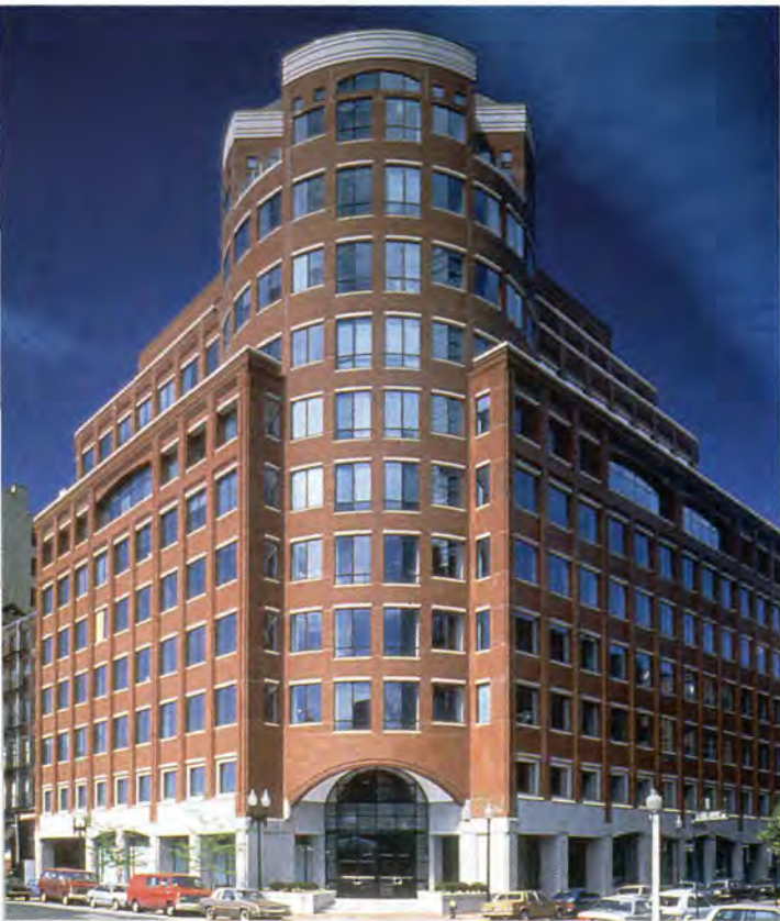
Fig. 6. Brick-clad precast concrete panels were used to speed up the construction time required for the 10-story office building at 745 Atlantic Avenue, Boston, Massachusetts. Corbeled brick, concrete sills and lintels, and recessed windows with arches continue the architectural vocabulary of the surrounding older buildings. Architect: The Stubbins Associates, Inc., Cambridge, Massachusetts.
