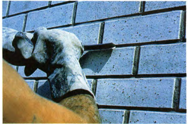
Fig. 20e. As the grout begins to set, the joints are tooled.
