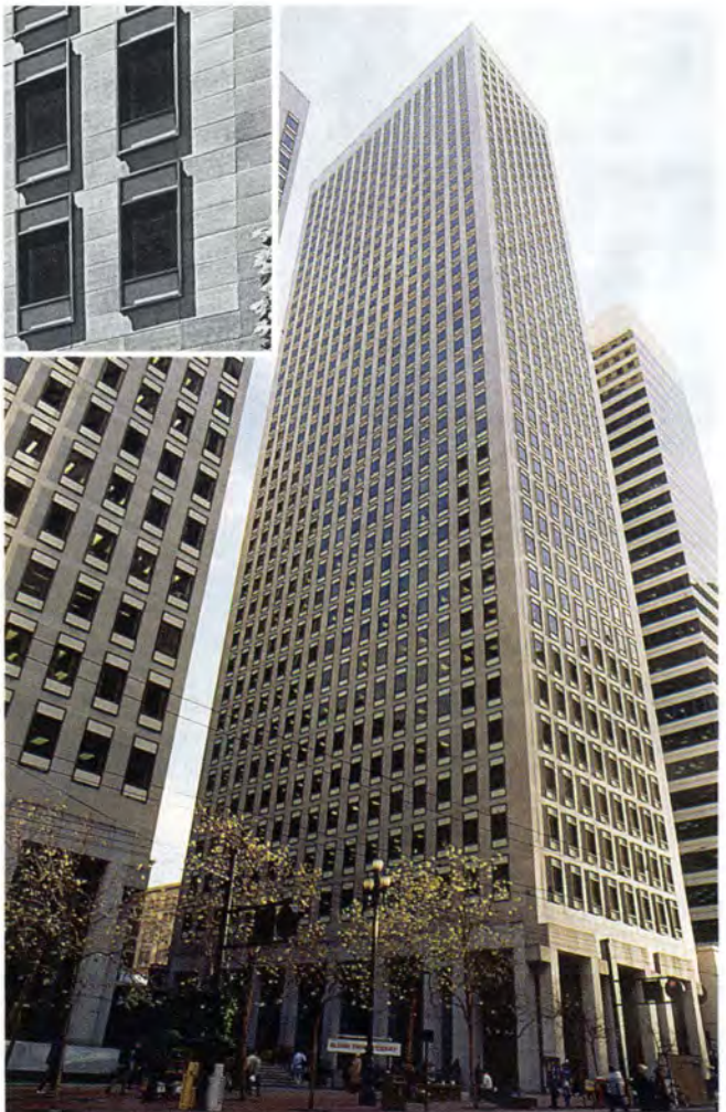
Fig. 11. This 42-story office building, 575 Market Street, San Francisco, California has 9 ft (2.7 m) wide by 13 ft (4 m) high L-shaped terra cotta-faced precast concrete panels. Seven equal 1 3/4 in. (44 mm) thick terra cotta pieces were placed in a structural lightweight concrete backup in the 7 1/2 in. (190 mm) thick story high panels. Architect: Hertzka & Knowles, San Francisco, California.
