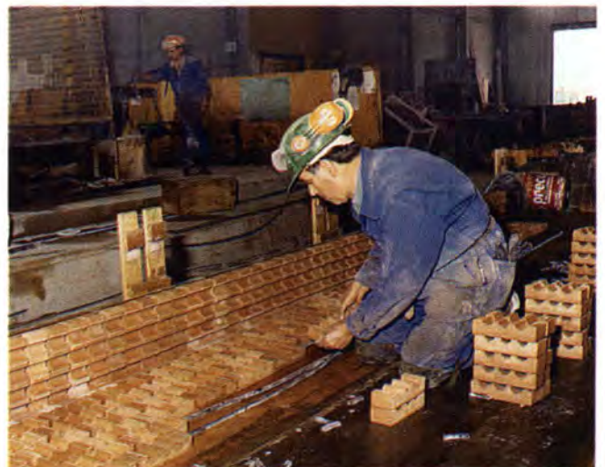
Fig. 14. Saw-cut bricks placed using loose rubber strips to separate the bricks.
