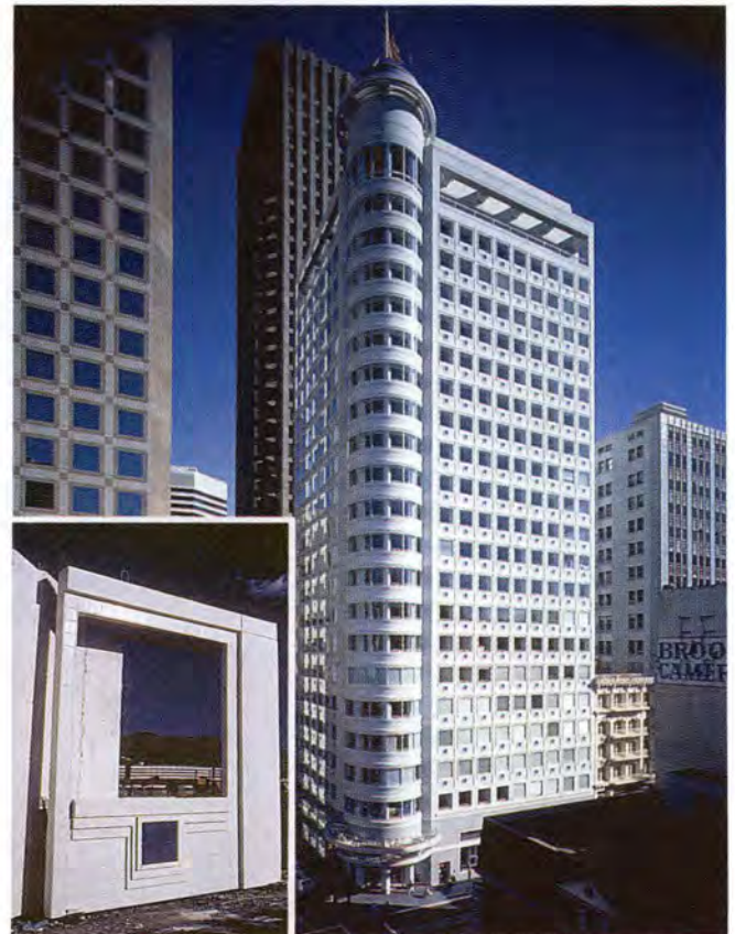
Fig. 8. The ability of architectural precast concrete to create the new and restore the old is demonstrated by the new 22-story San Francisco Federal Savings and Loan Building and (the barely visible) old six-story adjacent building (see Fig. 10). The 22-story tower has three different surface finishes: (1) lightly sandblasted white concrete, (2) 6 in. (150 mm) square glazed white ceramic tiles and some additional 10 in. (250 mm) square accenting blue tiles, and (3) a combination of the first two. Architect: Skidmore, Owings and Merrill, San Francisco, California.
