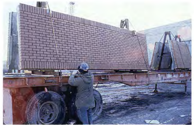
Fig. 18. Panel edges protected to prevent chipping during shipping.
