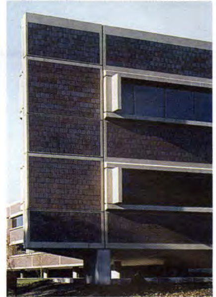
Figs. 9a and 9b. Spandrels and wall panels on Sylvan Corporate Center, Englewood Cliffs, New Jersey, have integrally cast 8 in. (200 mm) square brick-colored tiles with pigmented mortar. A beige band of concrete surrounds the tile field. Architect: Herbert Beckhard Frank Richlan & Associates, New York, New York.
