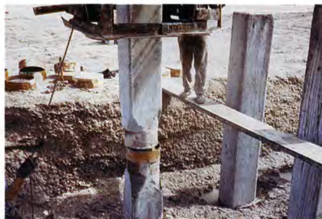
Fig. 2.13. Connector ring pile splice.
