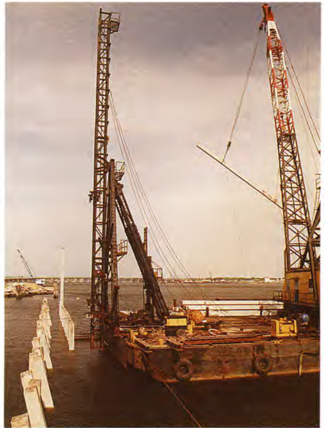
Fig. 2.2. Driving a batter pile to support a pier.
