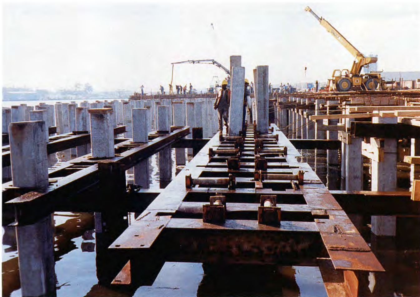
Fig. 5.1. Pile location established with the use of templates.
