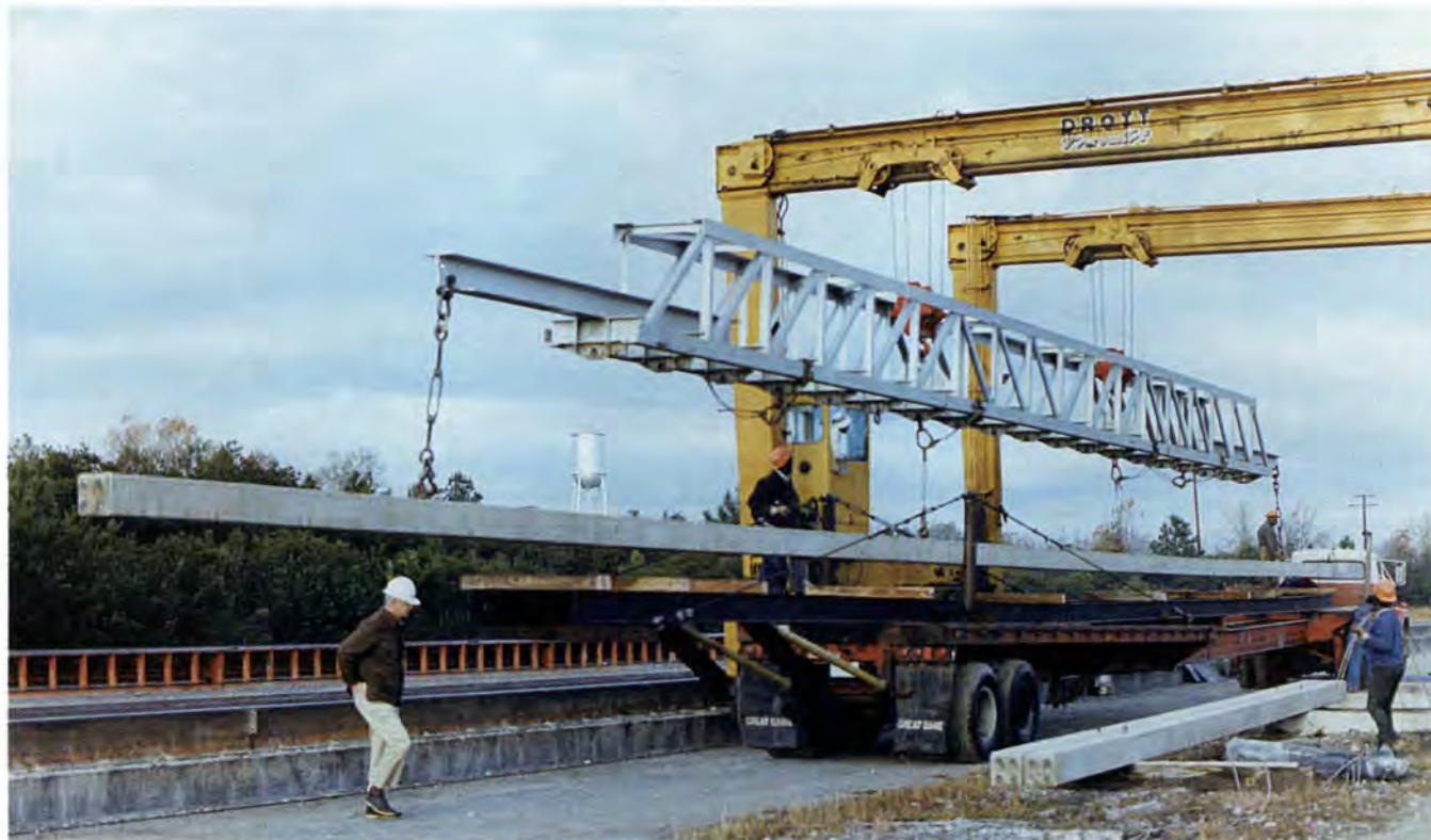
Fig. 2.1. Loading a 10 in. (254 mm), 113 ft (34.4 m) long prestressed concrete pile.
