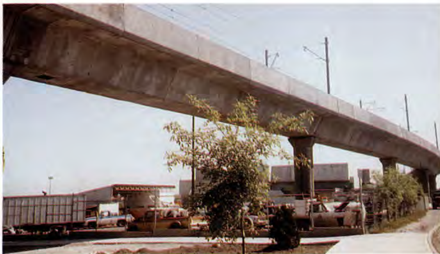
Fig. 25. A portion of the completed Metro line.
