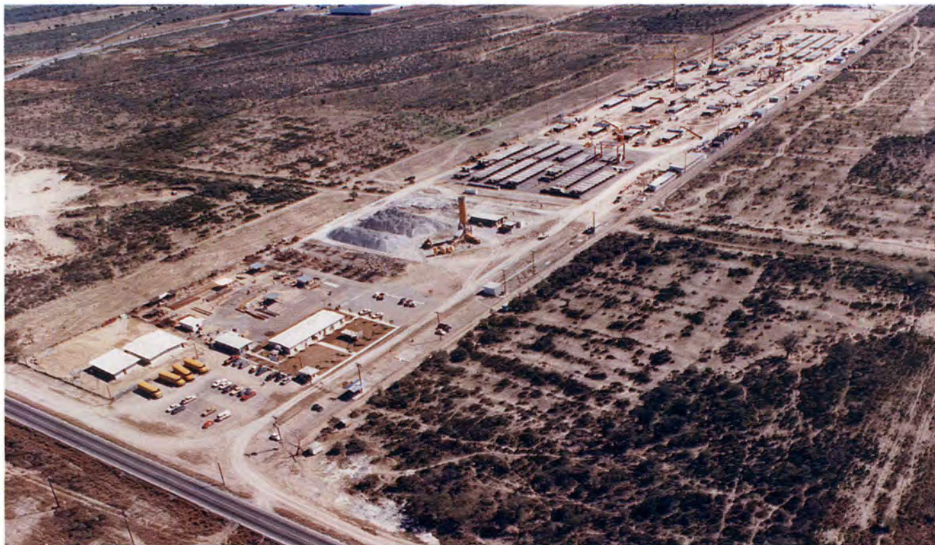
Fig. 10. Overall view of the large precasting plant located outside of Monterrey.
