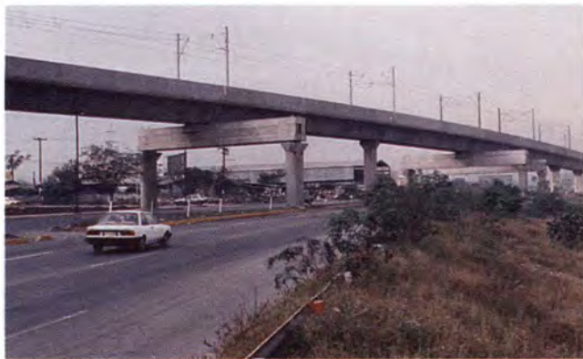
Fig. 8. Portion of completed structure showing use of straddle bents instead of single piers.
