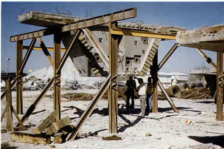
Fig. 16. Repair stand for correcting minor faults on completed segments.
