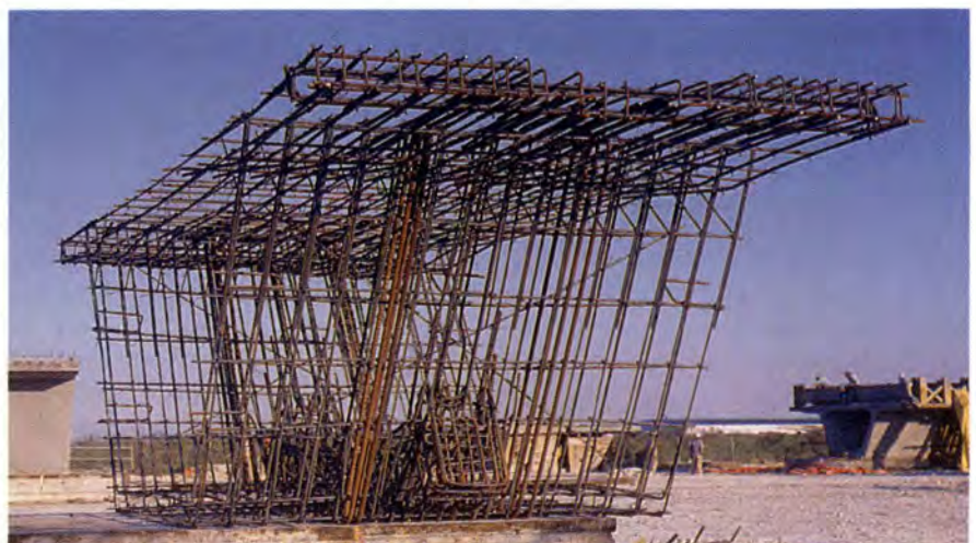
Fig. 12. Reinforcing bar cage for a typical segment.
