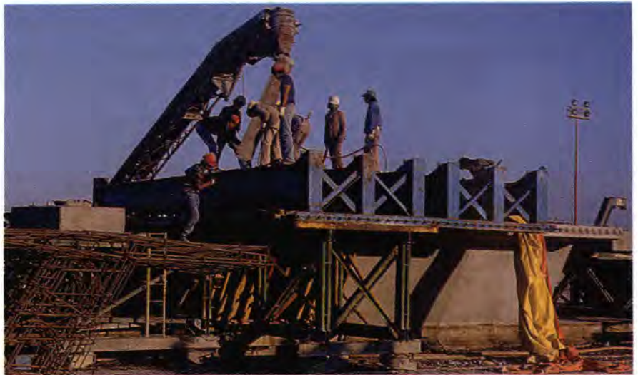
Fig. 13. A segment casting using a conveyor belt to move concrete from truck mixer to mold.
