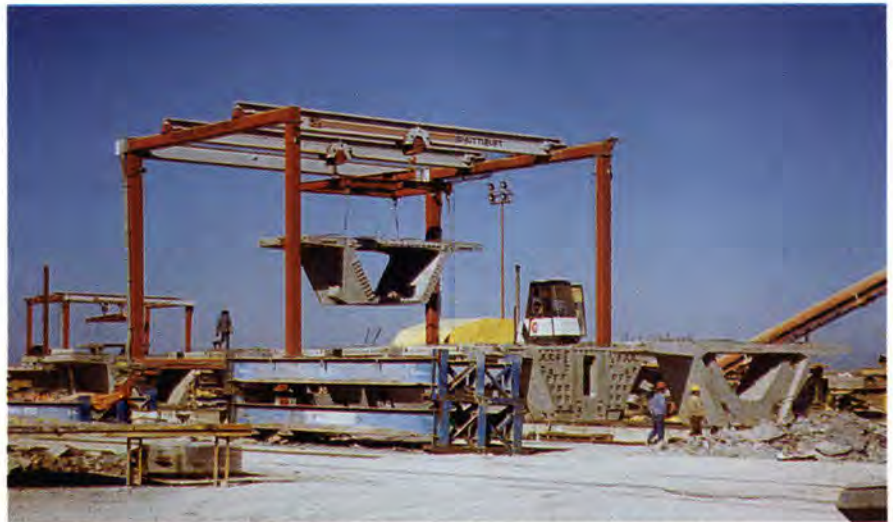
Fig. 14. Travelifts handle and transport completed segments in the plant.
