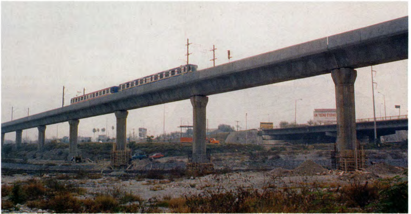
Fig. 1. A portion of the completed 18.7 km (11.6 mile) elevated Metro line for Monterrey, Mexico. All spans use segmental precast concrete construction.
