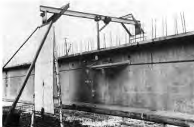
Fig. 24. King post bracing of a long prestressed concrete I-beam.
