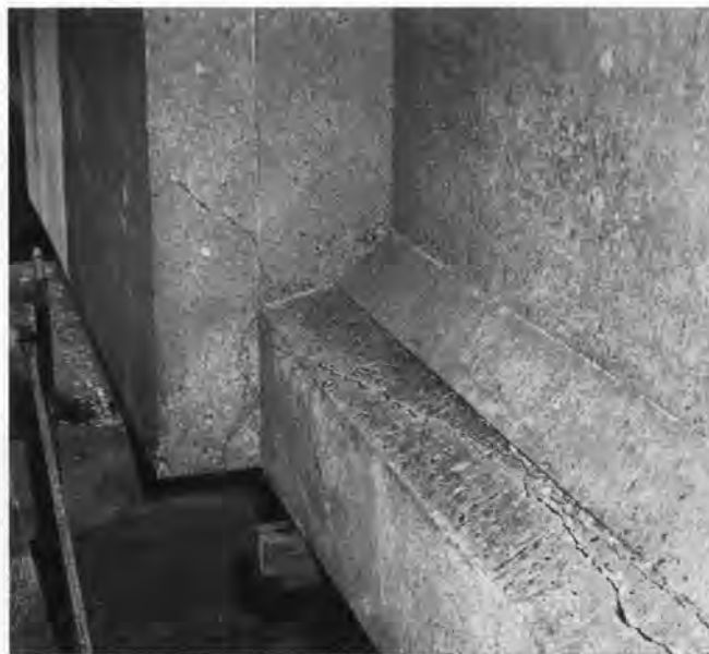
Fig. 18. New hairline diagonal crack appeared in end block of fascia girder.
