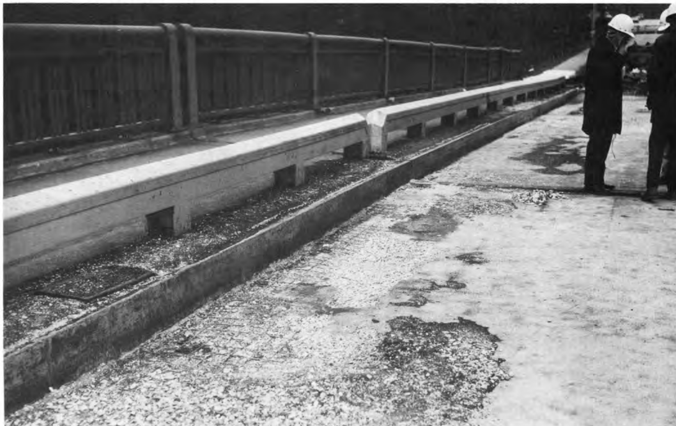
Fig. 15. Deterioration of concrete wearing surface in low point area of roadway, near joint.
