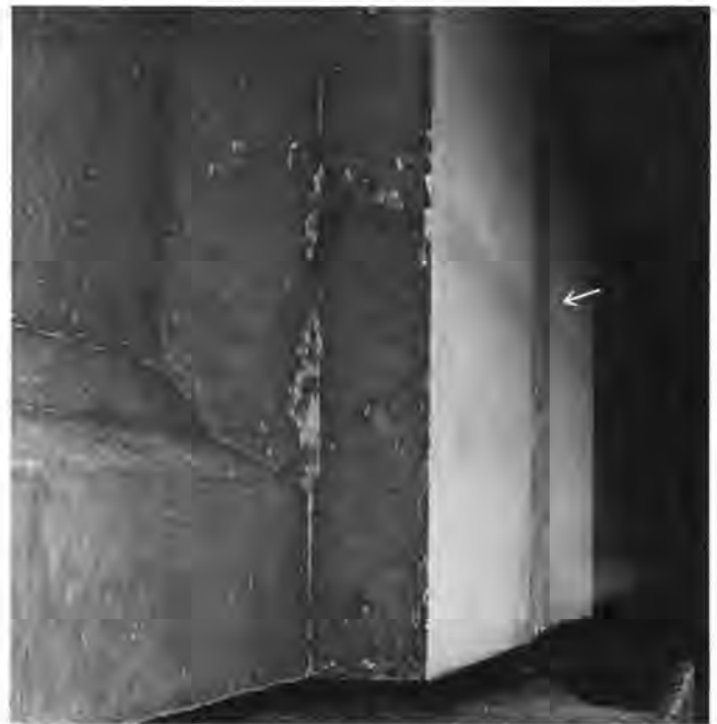
Fig. 19. Opened joint at contact between girder end block and cast-in-place concrete encasement protection over tendon anchorages.
