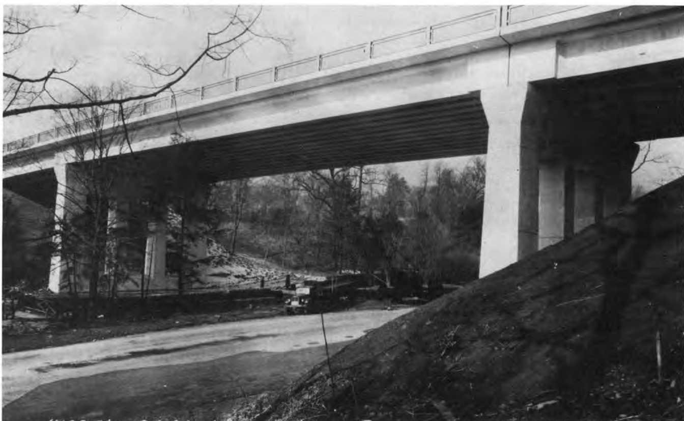
Fig. 12. Appearance of the south fascia girder after restoration and erection in 1950.
