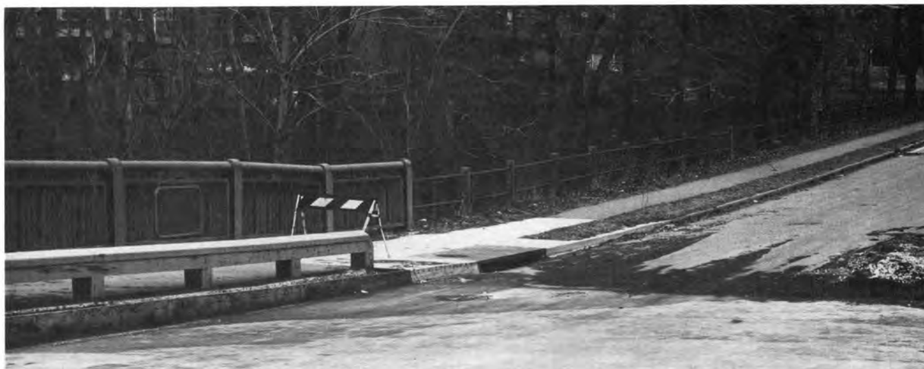
Fig. 16. Condition of abutment joint at roadway's low point, where water and snow collected. Note repair work.
