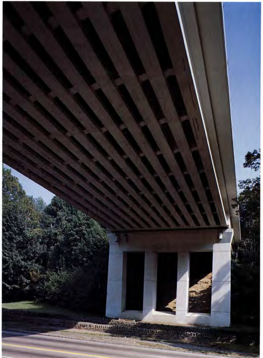
Fig. 1b. Underside view of Walnut Lane Memorial Bridge, showing post-tensioned I-girders. There were 13 such girders in the main span.
