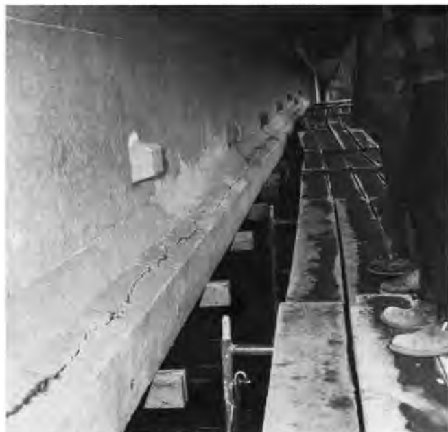
Fig. 13. Longitudinal crack in bottom flange of south fascia girder (1968).
