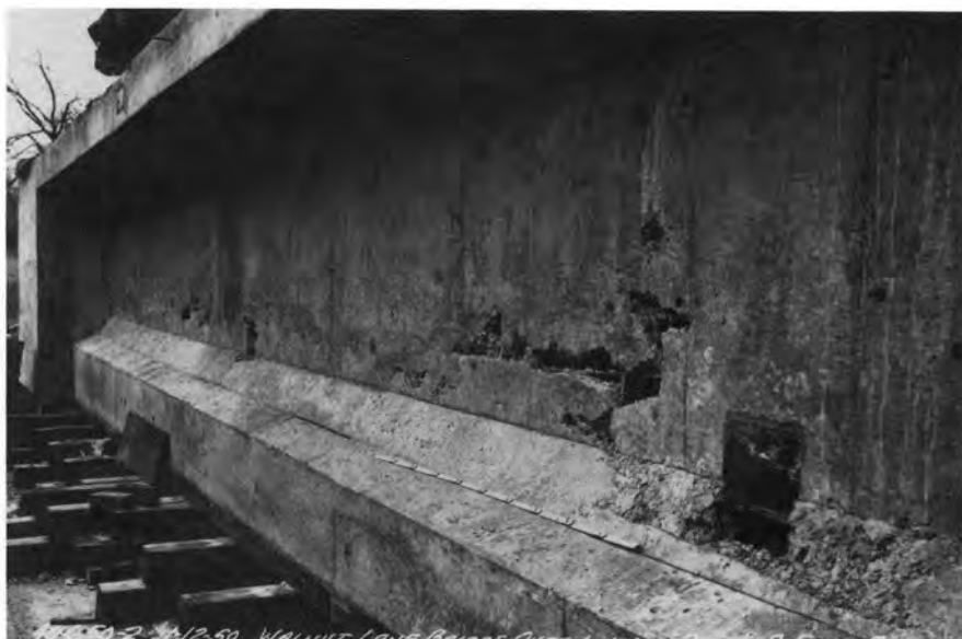
Fig. 11. Honeycombs in the first 160 ft (49 m) girder cast in 1949 for the Walnut Lane Memorial Bridge.
