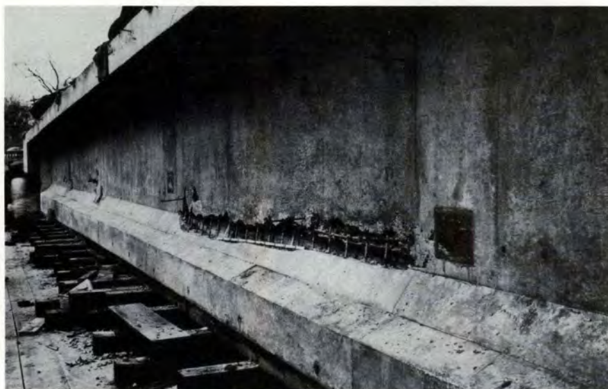
Fig. 10. Appearance of south side of first girder cast, after removal of forms. Note reinforcement displacement.
