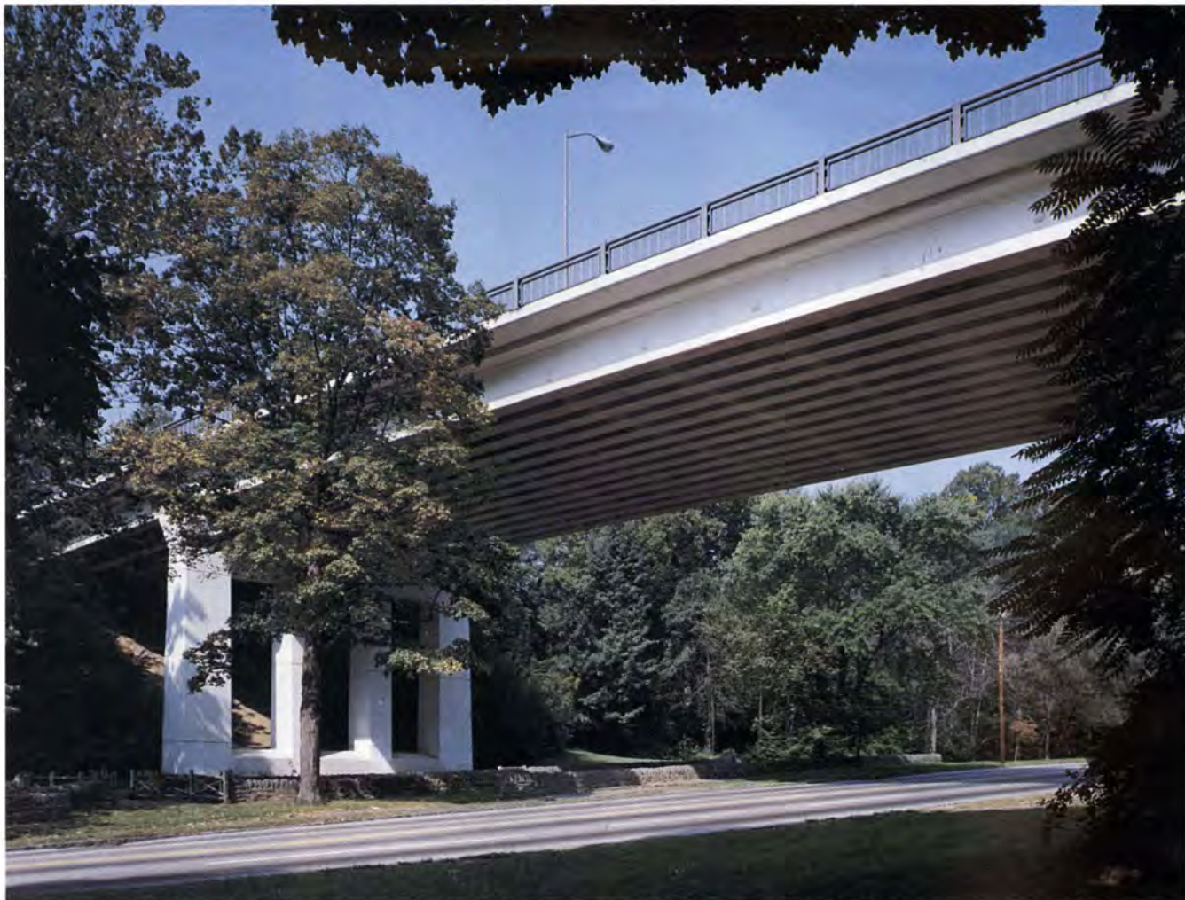
Fig. 1a. The original Walnut Lane Memorial Bridge in Philadelphia's Fairmount Park had a post-tensioned main span of 160 ft (49 m). The superstructure is about 50 ft (15 m) above Lincoln Drive.
