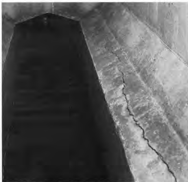
Fig. 17. Continued growth of major cracks noted in the 1970s.
