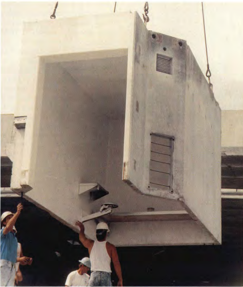
Fig. 9. Finished cell ready for shipping.
