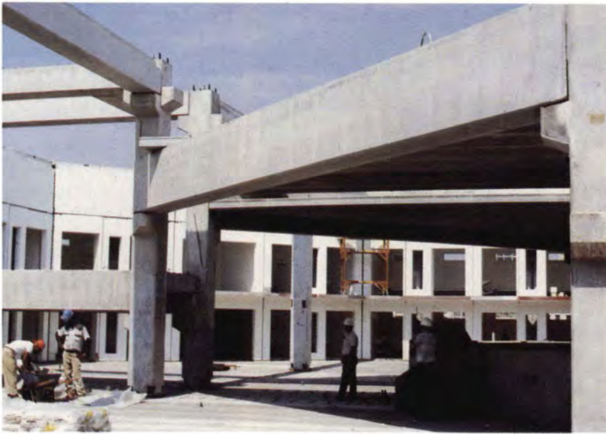
Fig. 11. Column-to-beam framing arrangement.
