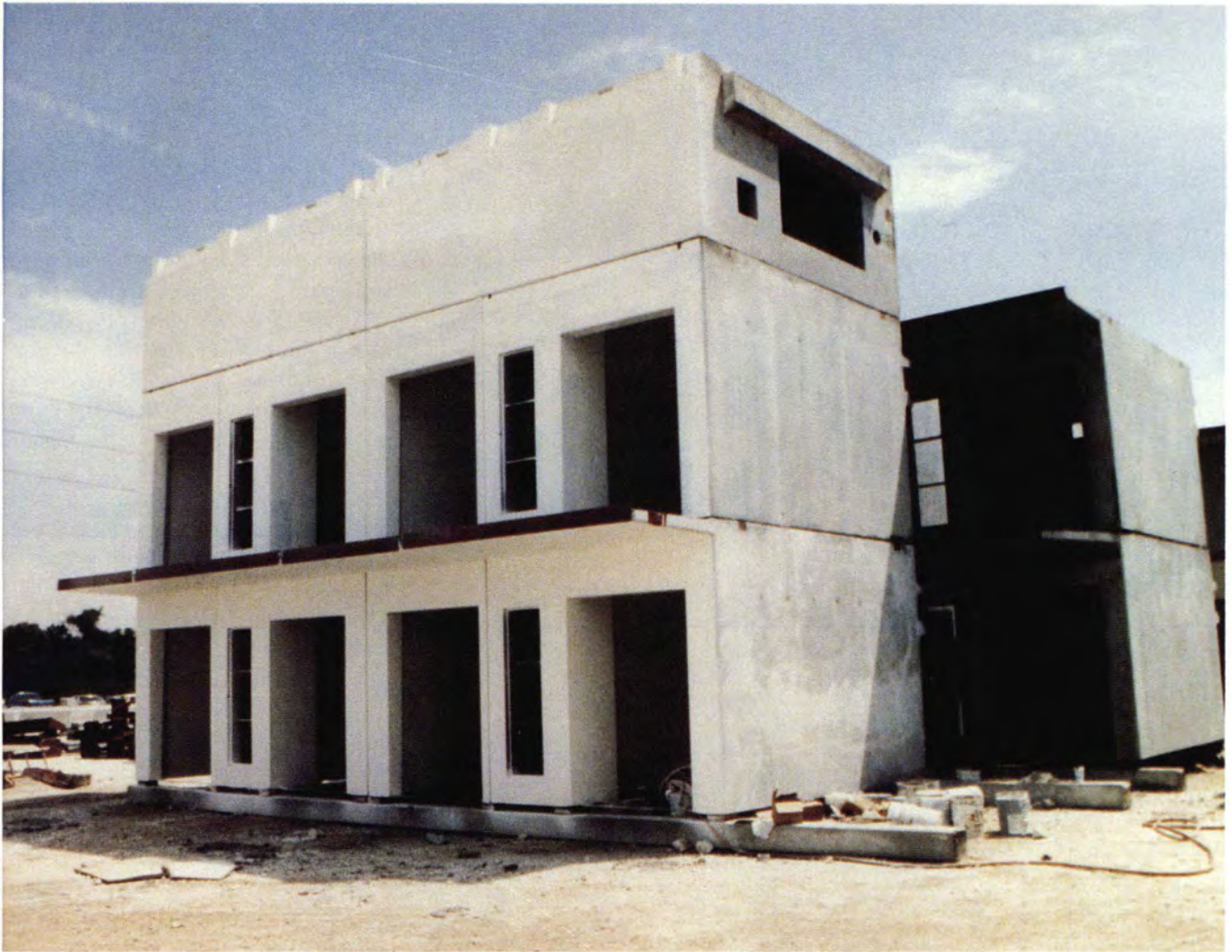
Fig. 5. Cell "three-pack" assembly in plant.
