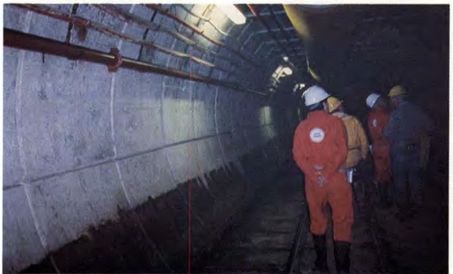
Fig. 3. Erected tunnel liners, Eurotunnel project.
