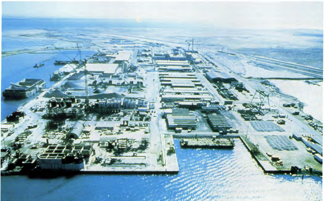
Fig. 4. Precast concrete production plant for King Fahd Causeway Bridges, Saudi Arabia to Bahrain.
