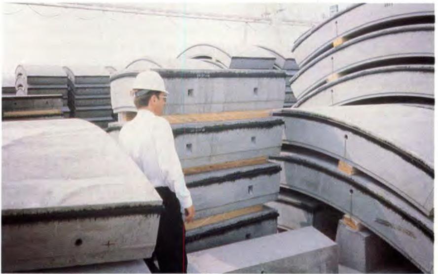
Fig. 2. Extremely close tolerances are demanded for tunnel liners.
