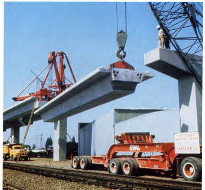
Fig. 7. Post-tensioned girder for BARTD Metro System, San Francisco, California.
