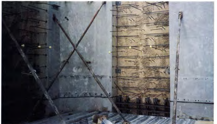
Photo 9. Interior elevation detail at tower shaft illustrates the back of veneer precast panels and exposed reinforcing bars of structural precast panels. This space will be filled with cast-in-place concrete.
