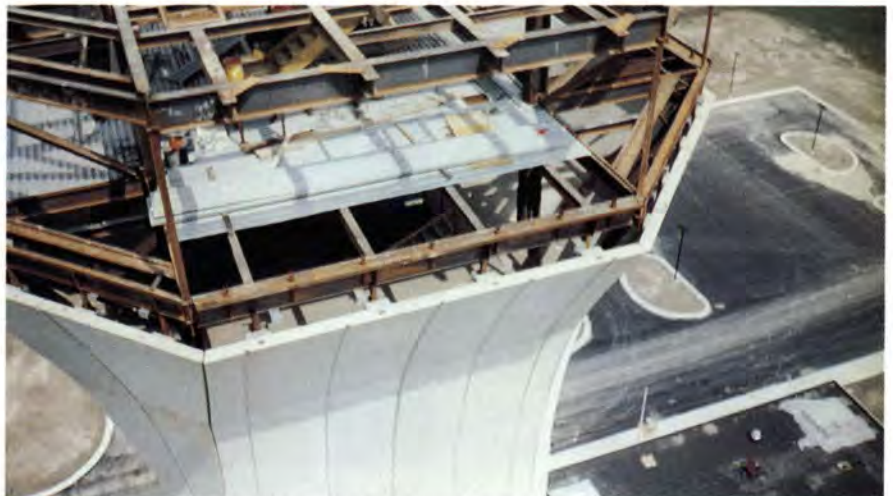
Photo 10. Tower shaft at 199 and 186 ft (61 and 57 m) level showing flare of precast panels.
