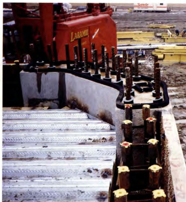
Photo 4. Rubber gasket around perimeter of horizontal joints.
