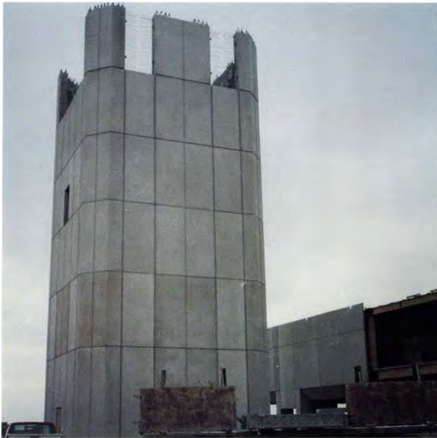
Photo 6. Tower shaft showing structural precast panels shored in place. Base building at right is clad with architectural panels.
