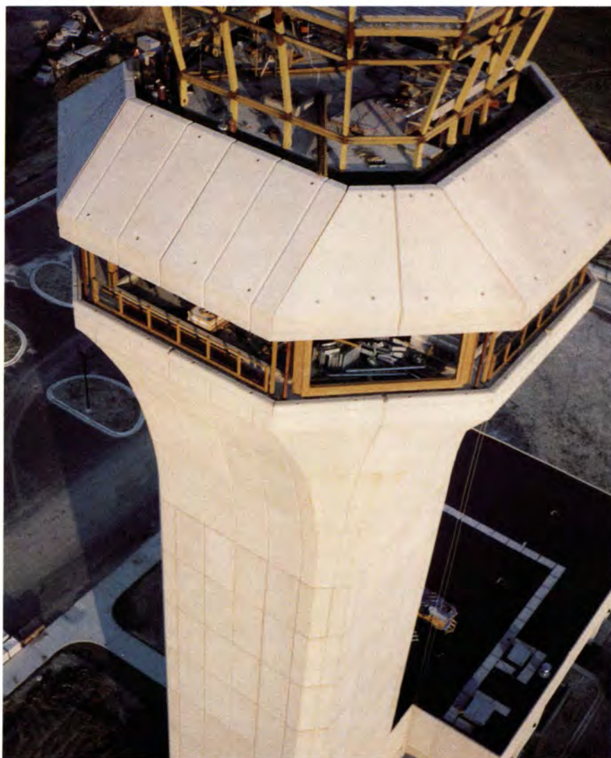
Photo 13. Aerial view of precast concrete tower with base building below it. The tower shaft is structural precast concrete while the upper flared portion and cap is architectural precast concrete.
