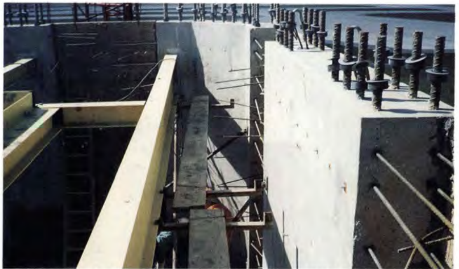
Photo 8. Detail at structural precast panels showing horizontal reinforcing bars extending into void space where cast-in-place concrete tie panels together. Note that vertical reinforcing bars will extend into splice sleeves.
