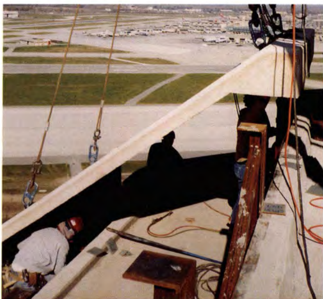
Photo 11. Erection of architectural precast panel at top of tower.
