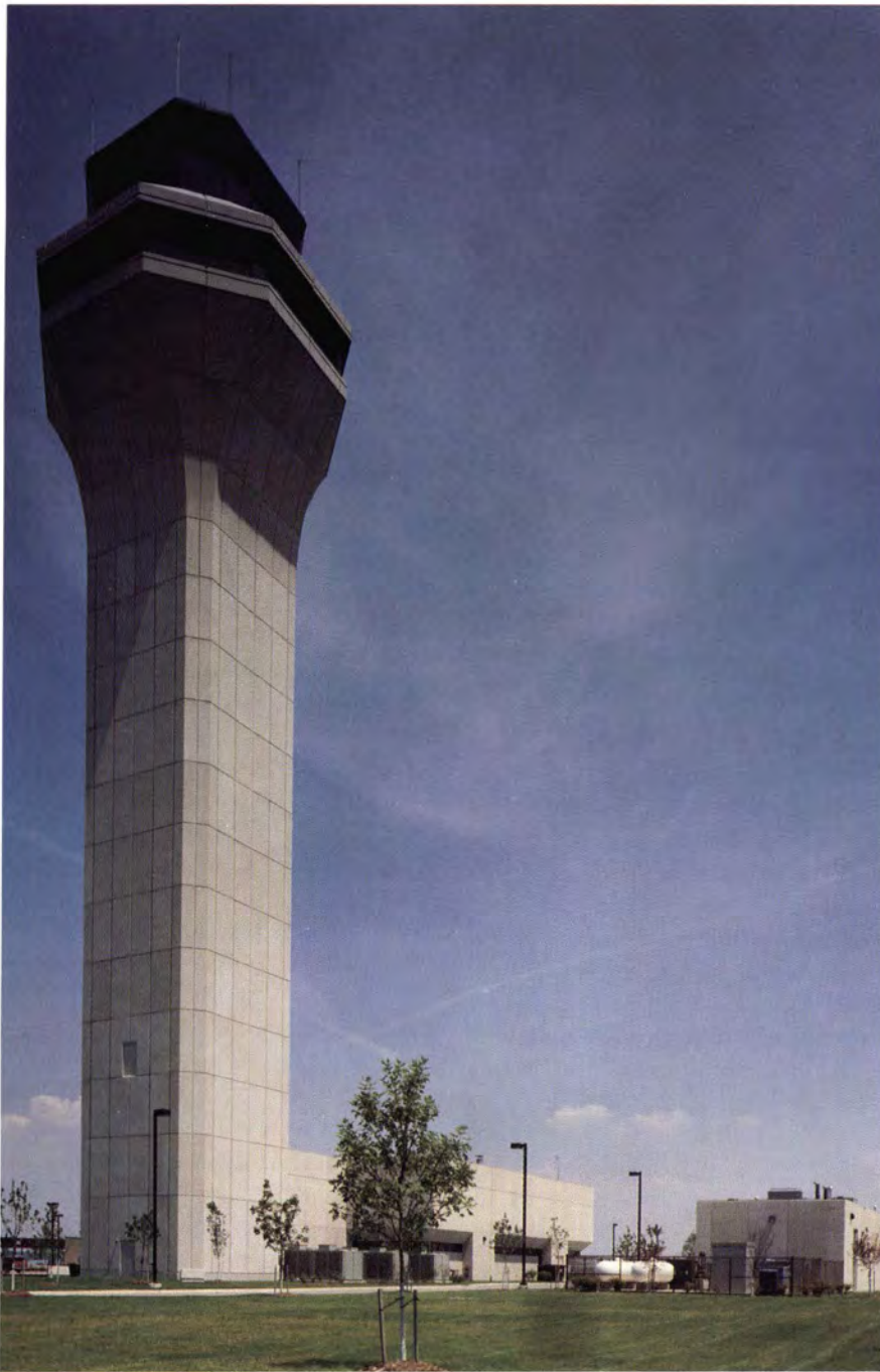
Photo 15. West elevation of completed air traffic control tower, base building and auxiliary utility building.
