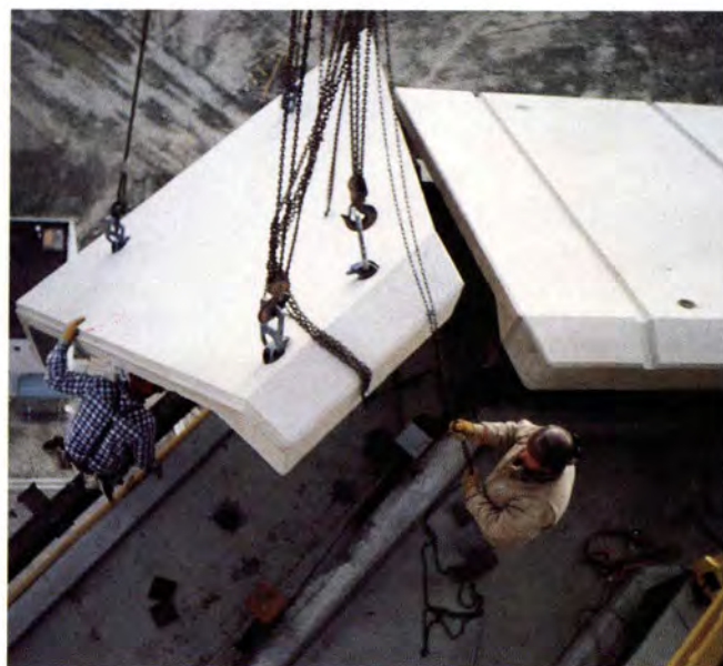
Photo 12. Erection of architectural precast panel next to in-place panels.
