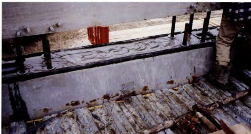
Photo 5. Grouted horizontal panel joint ready to receive panel above it.
