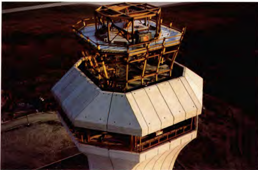
Photo 14. Top portion of control tower. Architectural precast panels are clad on a steel frame. The remaining areas are enclosed with glass, metal insulated panels and microwave transparent fabric.
