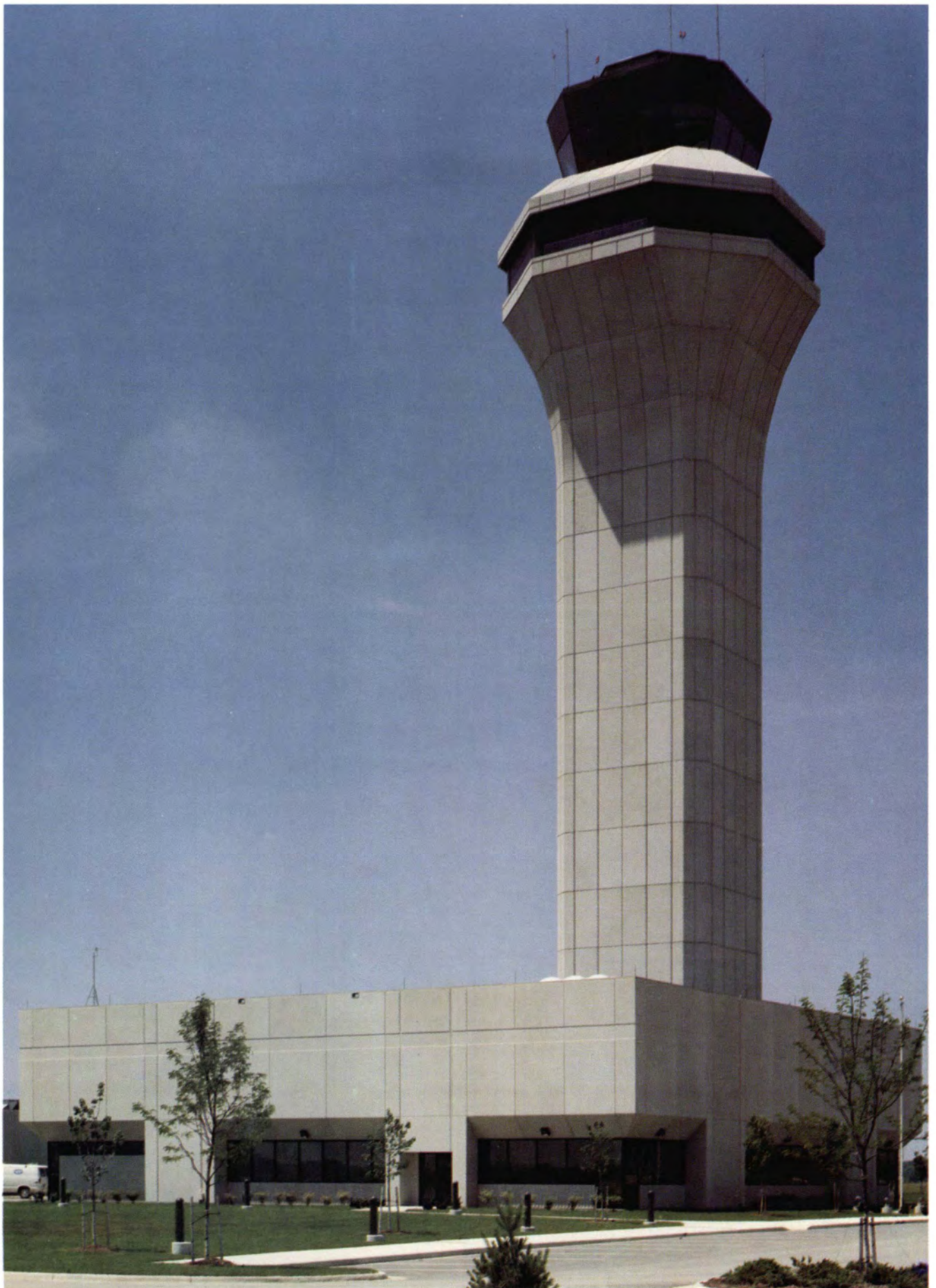
Photo 1. East elevation of completed air traffic control tower and base building.
