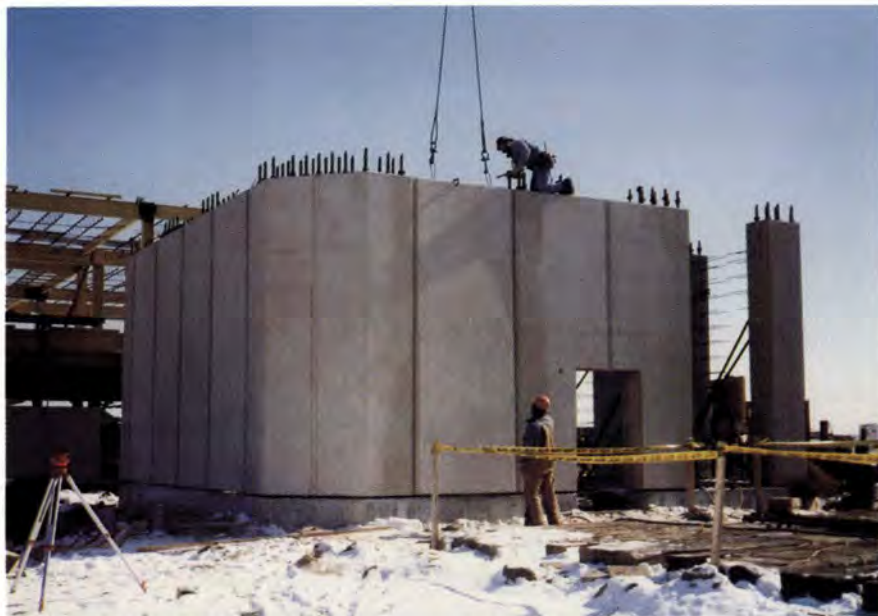
Photo 2. Erection of first level panels looking from west.
