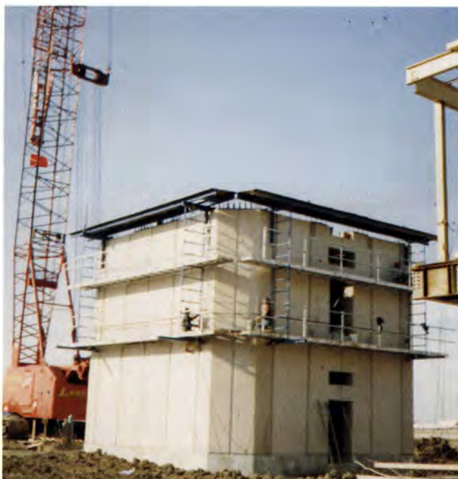
Photo 3. First level panels looking from east. Exterior scaffolding was used in grouting horizontal joints and splice sleeves.
