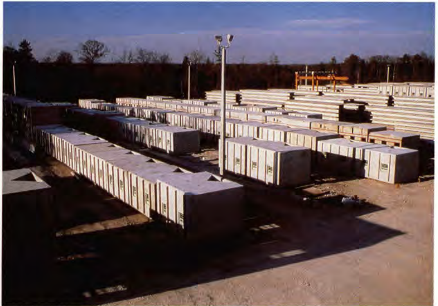
Cell units in yard awaiting erection.
