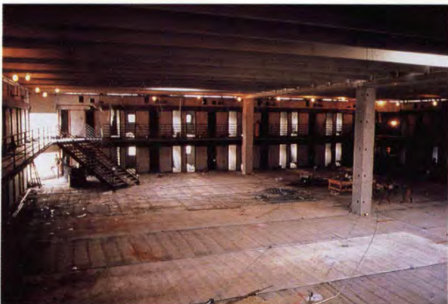
At left is the unfinished dayroom interior. At right is the finished dayroom interior. Long span prestressed double tees allowed for open dayrooms which facilitate observation by control room guards.
