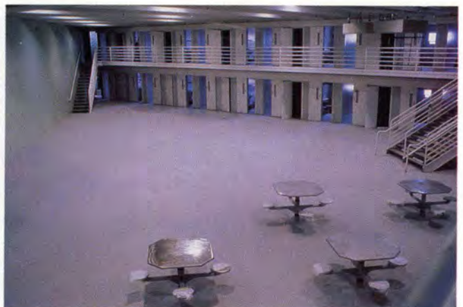
At left is the unfinished dayroom interior. At right is the finished dayroom interior. Long span prestressed double tees allowed for open dayrooms which facilitate observation by control room guards.
