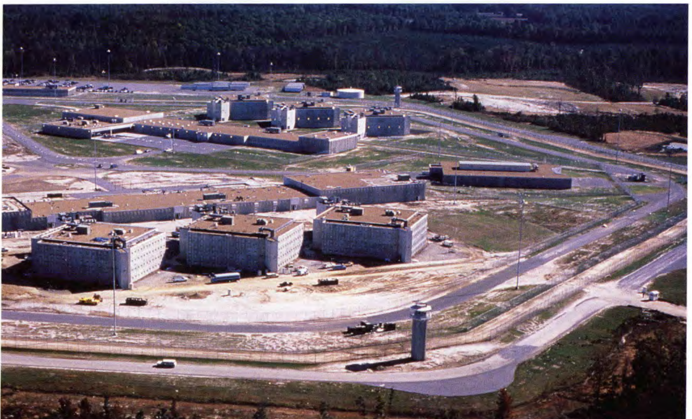
Aerial view showing three housing buildings. Note that three 176-cell housing buildings and program support building comprise one prison unit.
