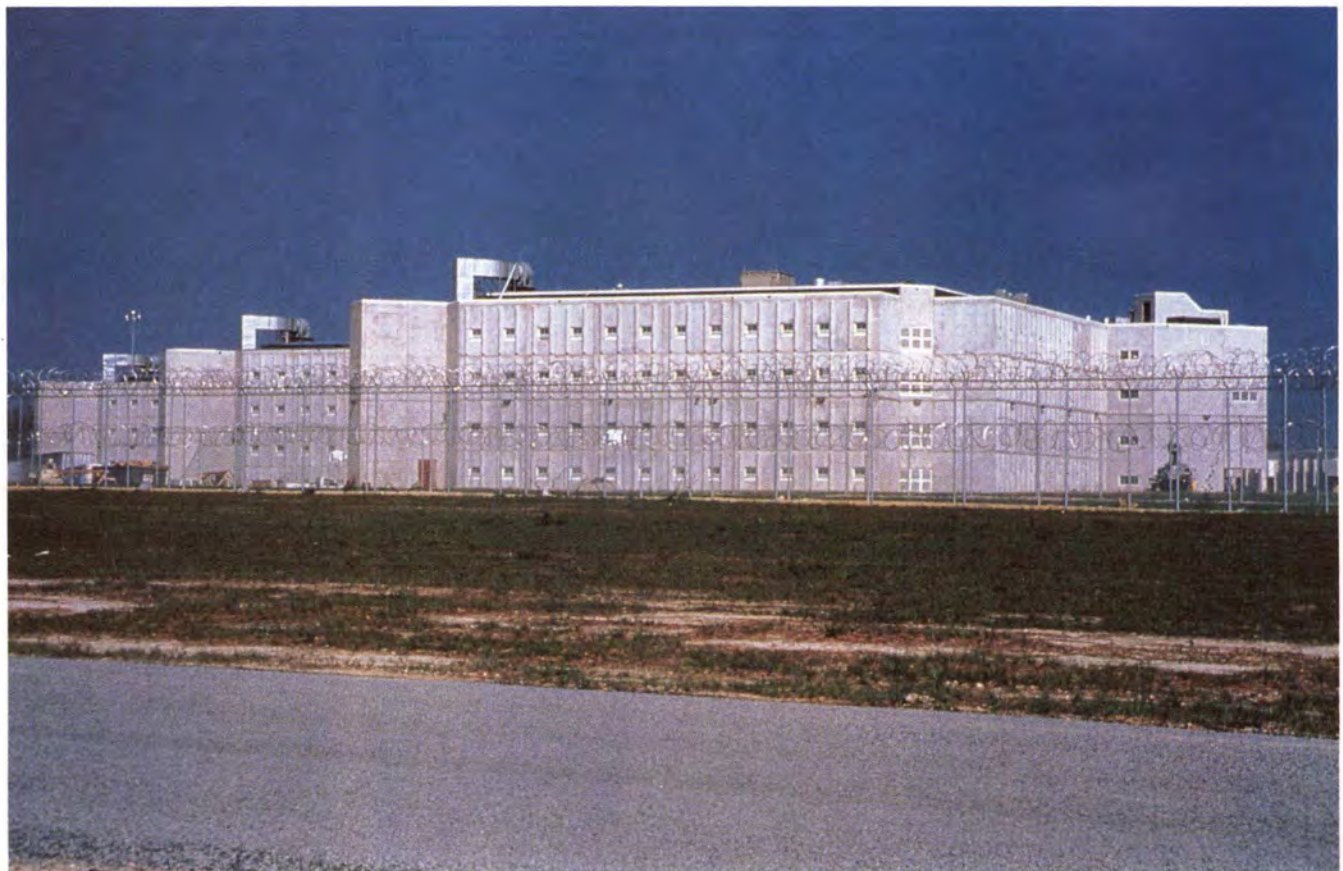
Elevation of housing with security fence.
