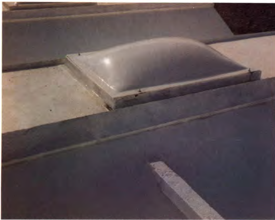
Fig. 29. Skylight window developed for roof systems in Honduras.
