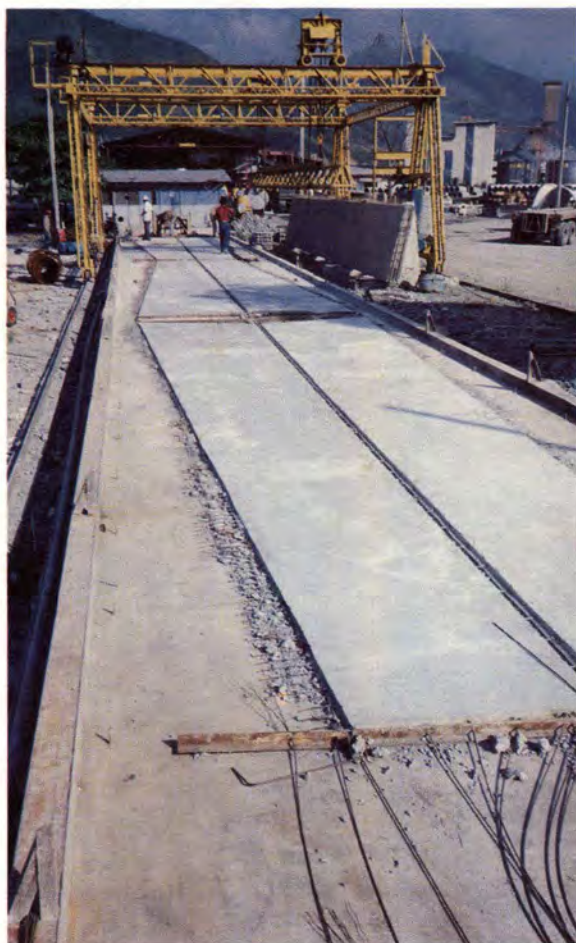
Fig. 3. Self-stressing steel form used for V-plate fabrication.
