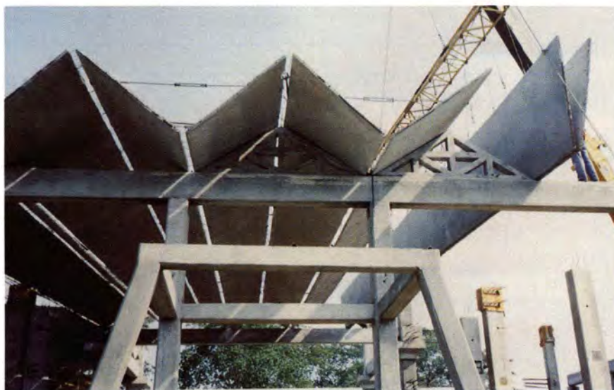
Fig. 6. Tapered V-plate roof elements during erection of the Good Shepherd Catholic Church.
