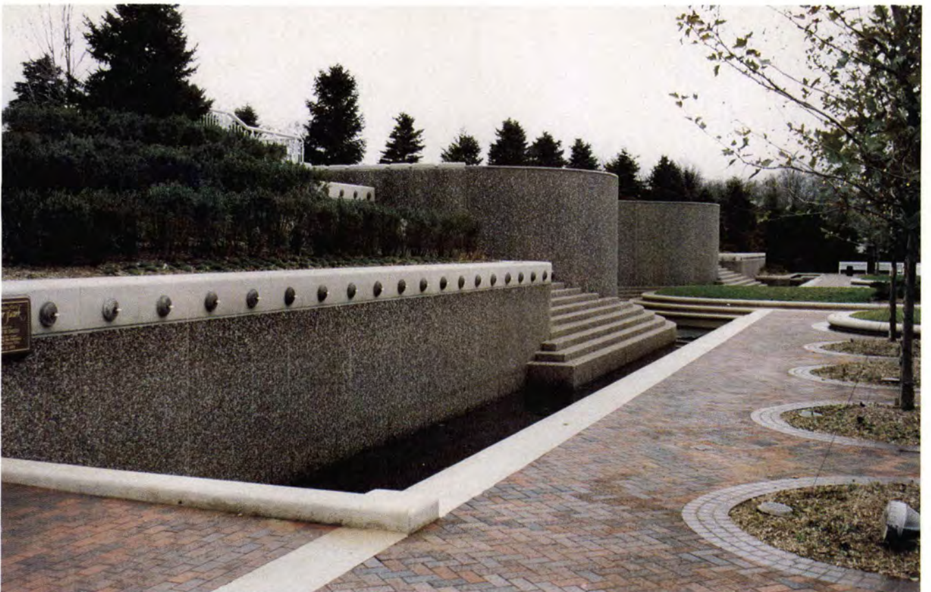
Fig. 8. View of lower pool/perimeter wall (north end).
