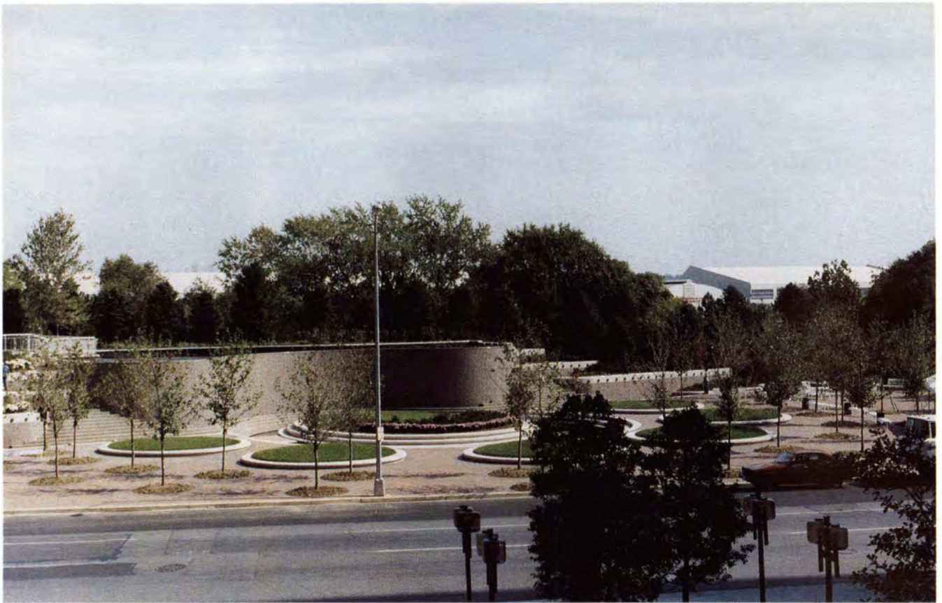
Fig. 6. View from the west.
