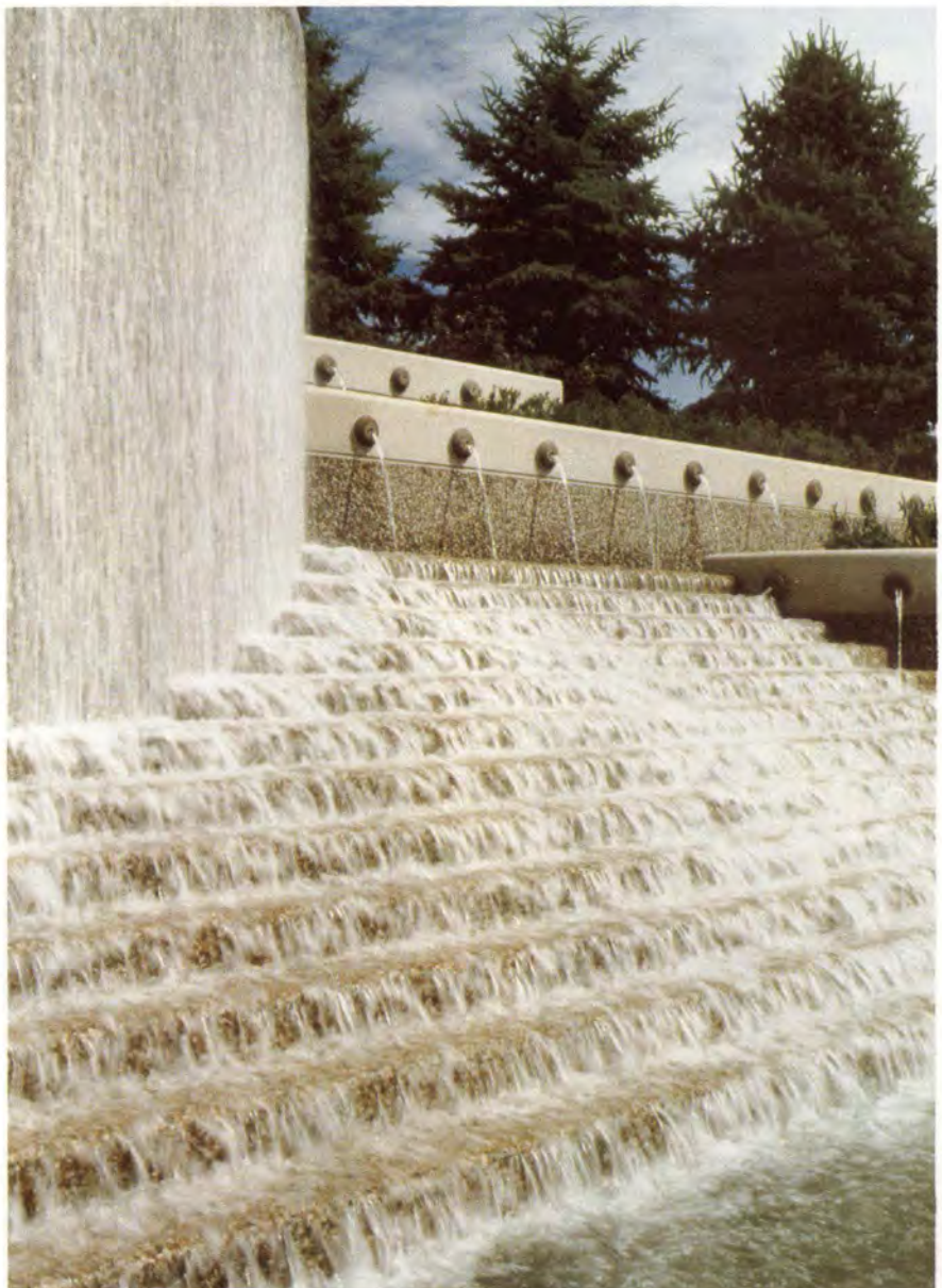
Fig. 3. Detail of steps (south end).
