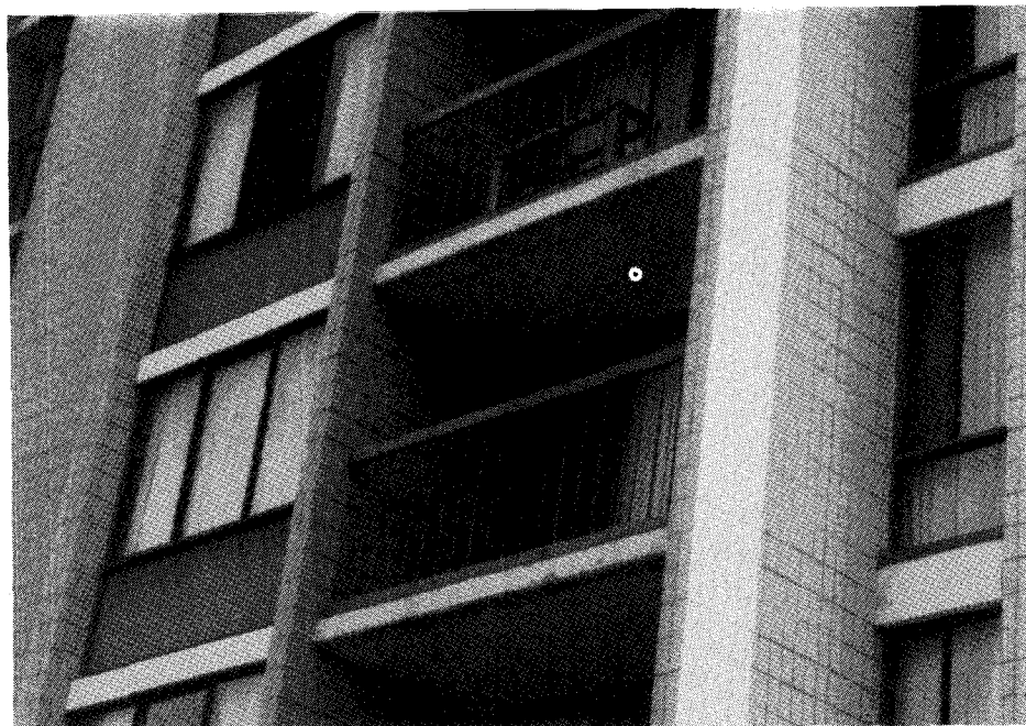
Fig. 16. Closeup of hollow-core balcony.
