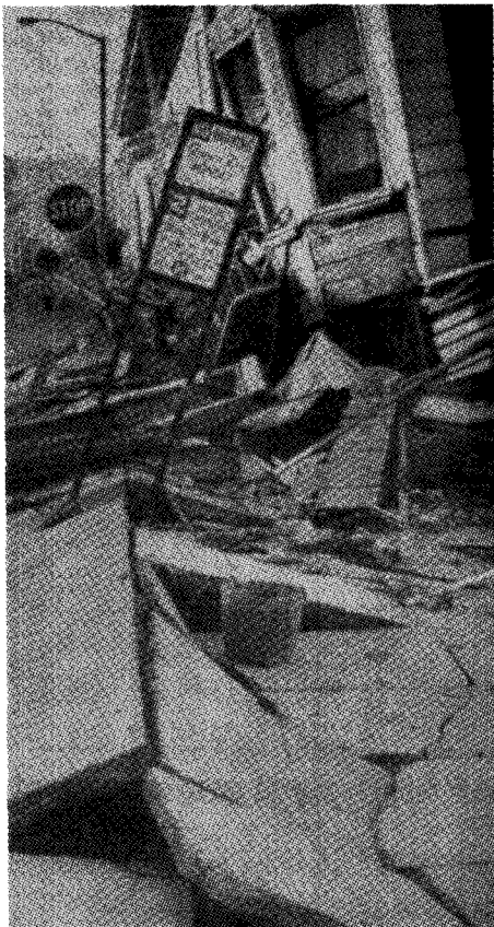
Fig. 5. Damage to homes and pavement in the Marina area of San Francisco.
