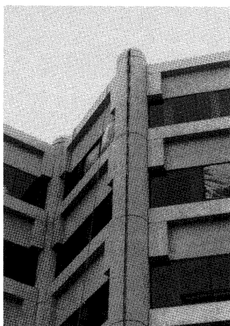
Fig. 11. Opened seismic joint.
