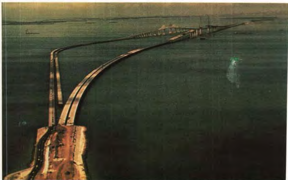
Fig. 1. A finished view of the new bridge with old bridges in the background. This is the first time a major crossing has been designed for ship impact along its entire span.
