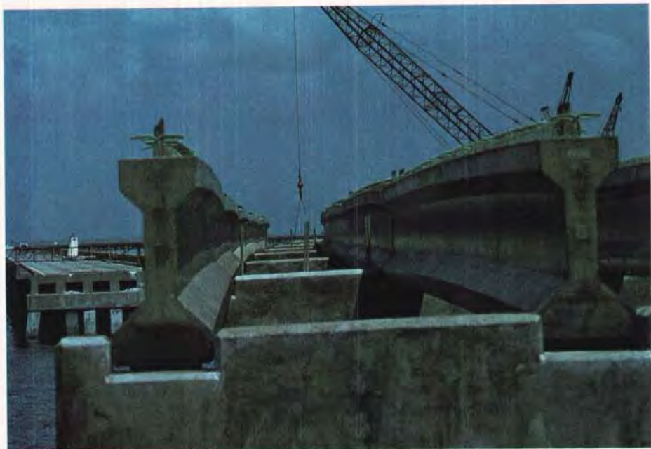
Fig. 21. Precast prestressed concrete beams after erection.
