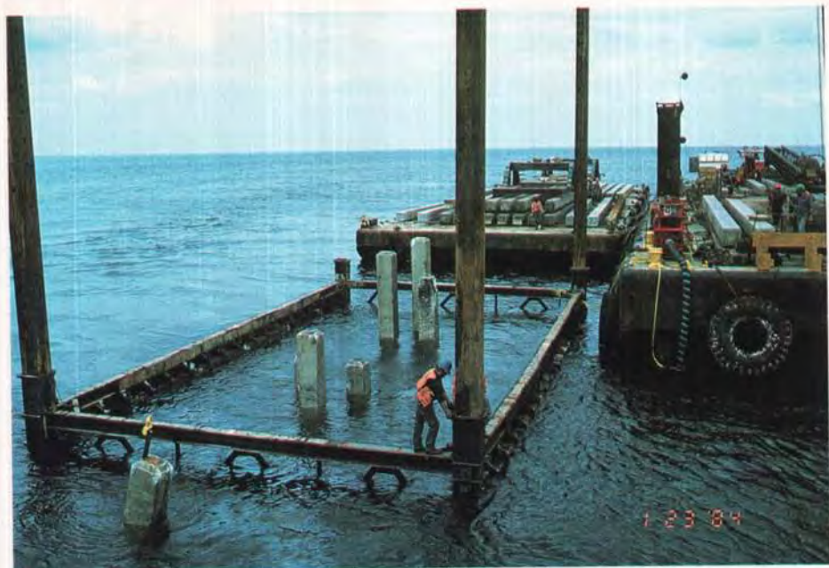
Fig. 6. Precast prestressed concrete piles being driven using template.
