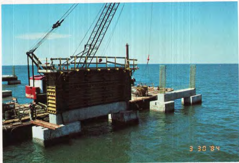
Fig. 18. Pile caps after construction.
