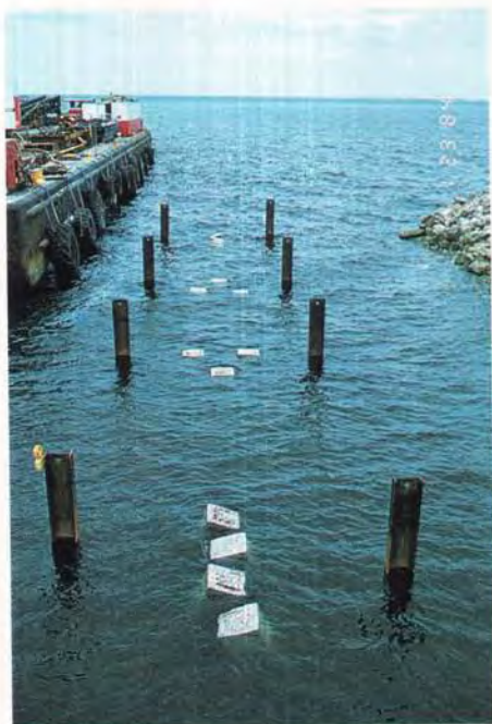
Fig. 7. View of precast prestressed piles after cut-off.
