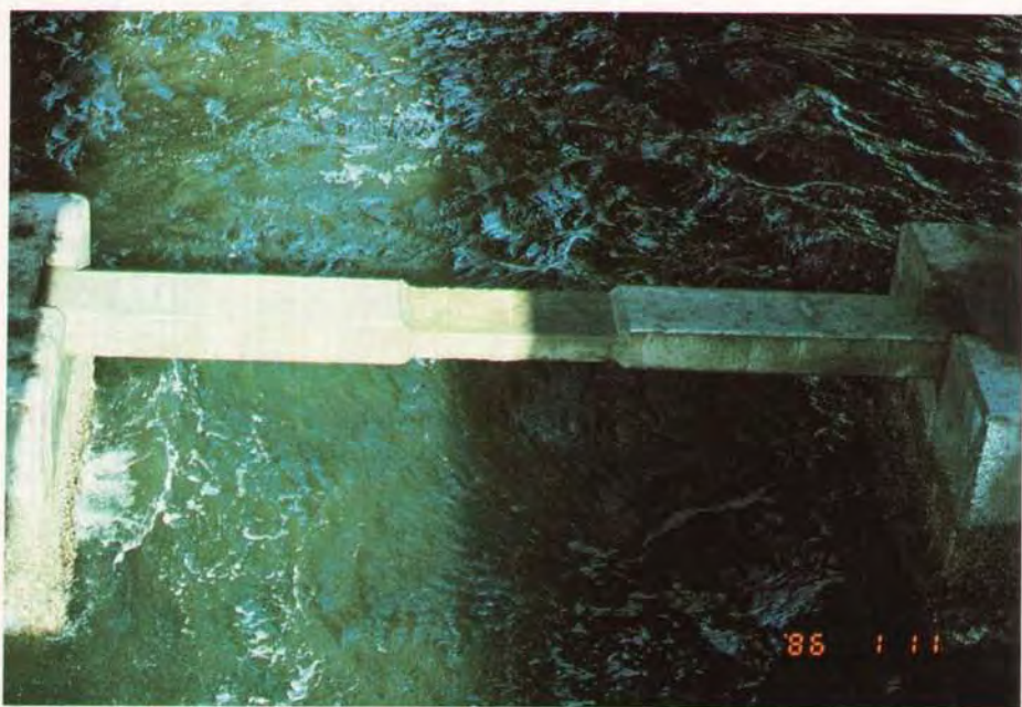
Fig. 24. Precast prestressed concrete frangible strut in place.
