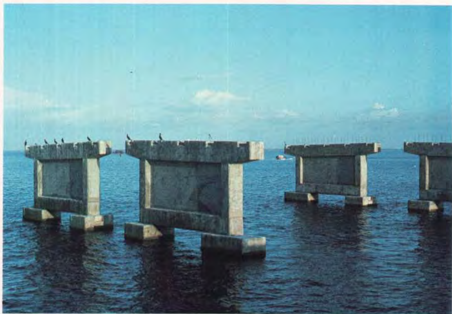
Fig. 20. Piers after construction.
