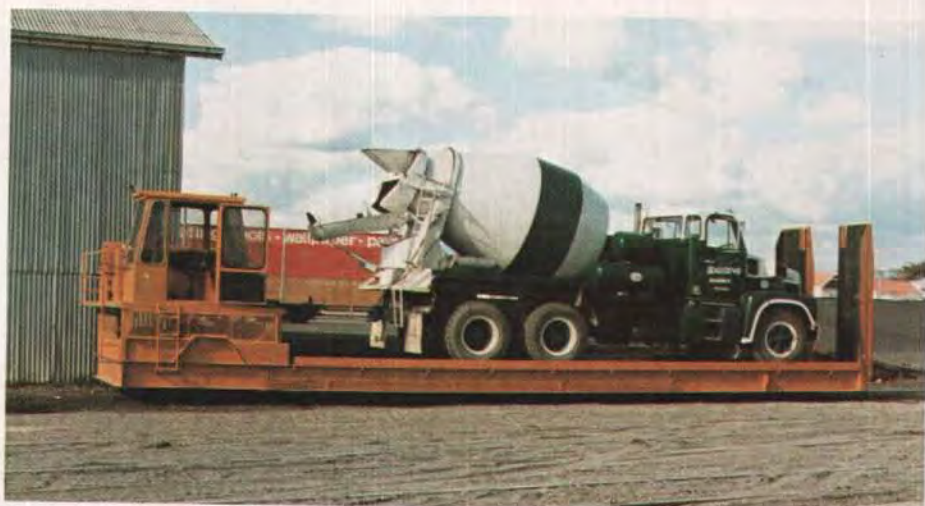
Fig. 4. Rail mounted concrete transporter for casting in place pole foundations.
