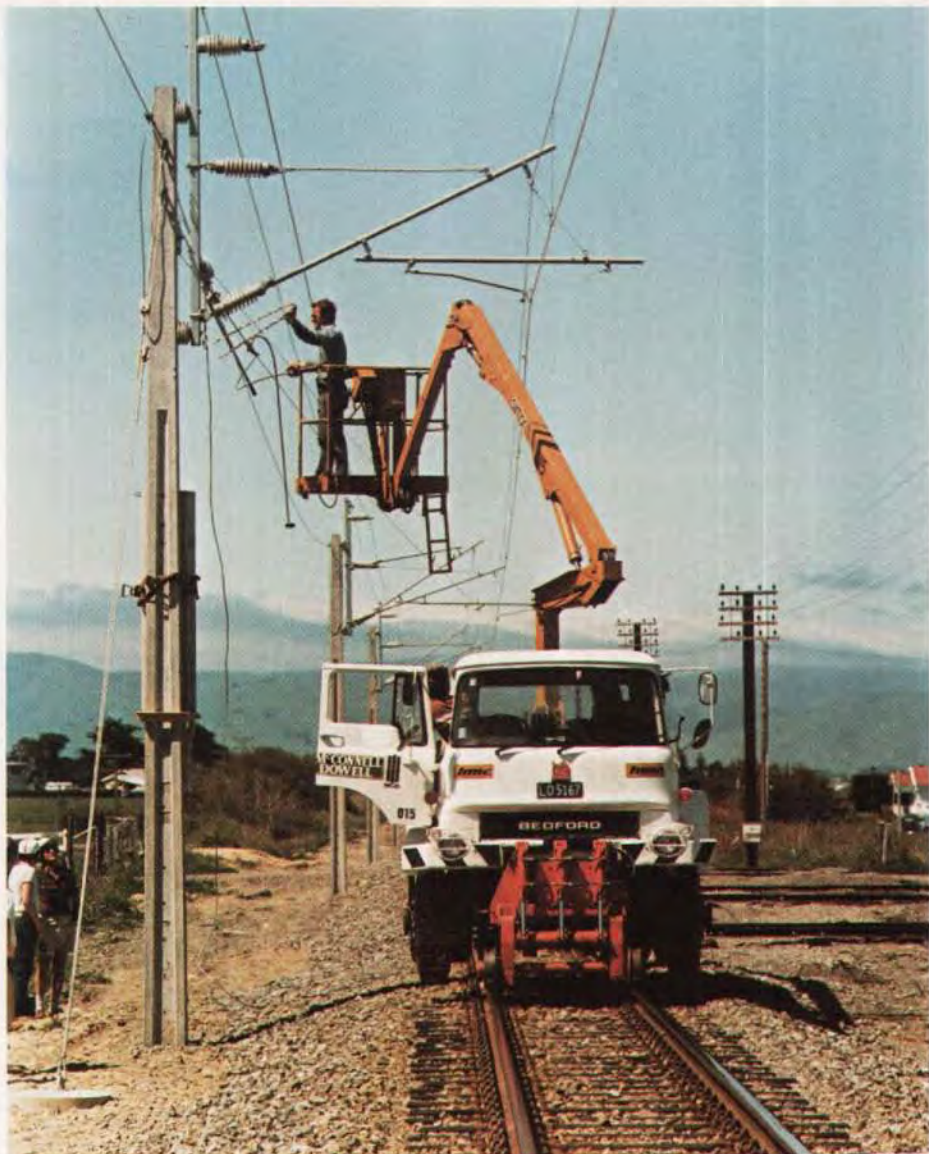
Fig. 6. Hi-Rail truck with hydraulic lift platform installing conductors.
