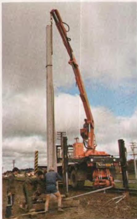
Fig. 3. Pole installation using rail mounted crane.
