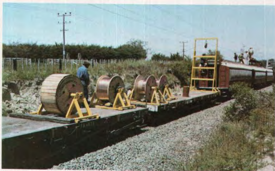
Fig. 5. Equipment used for running out the contact wire.
