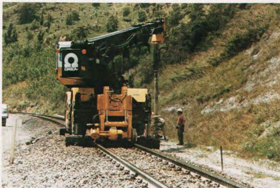
Fig. 2. Hi-Rail crane with auger attachment prepares to excavate a pole foundation.
