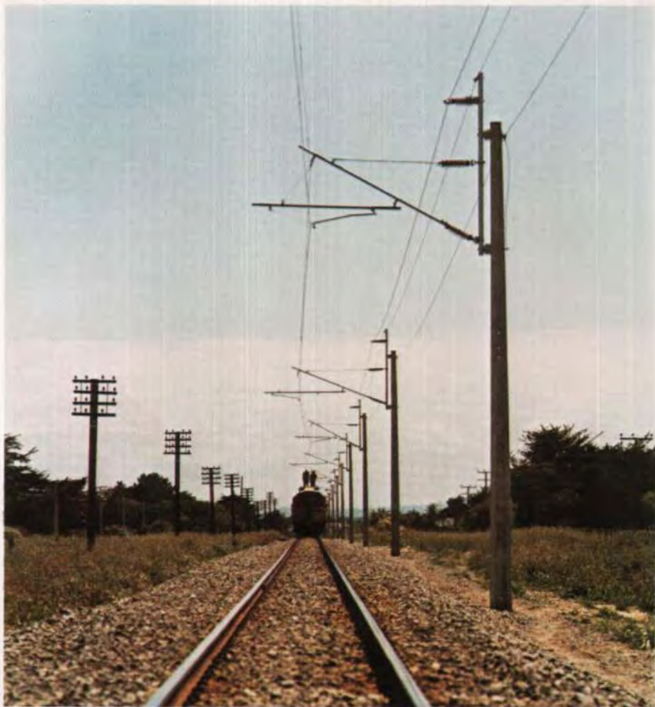
Fig. 7. Final adjustment of contact wire showing finished pole configuration.
