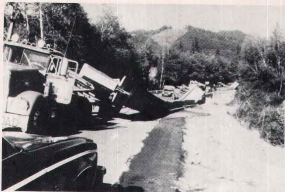
Fig. 7. Collapse of long span beam.
