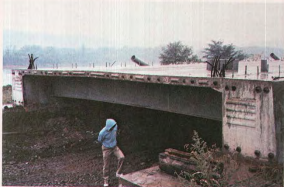
Fig. 6b. Casting bed arrangement of precast segment.
