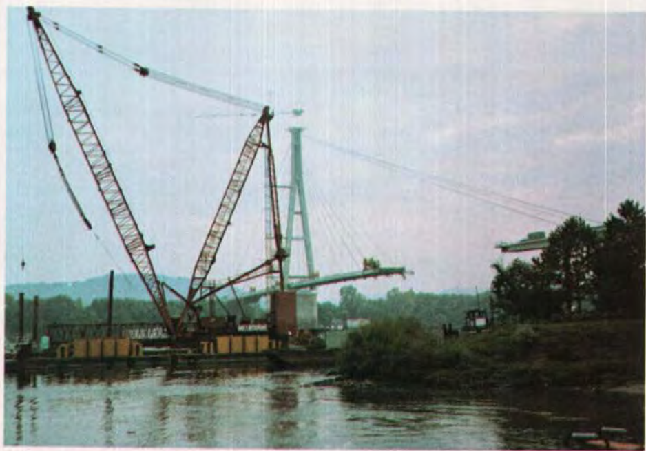
Fig. 7. Barge crane for segment erection.
