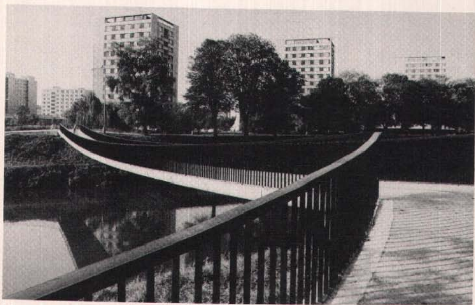
Fig. 3. Pedestrian bridge at Kromeriz.
