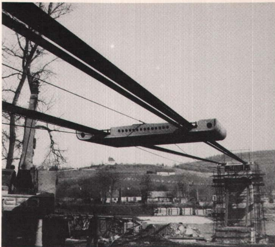
Fig. 10. Typical precast segment on bearing cables.
