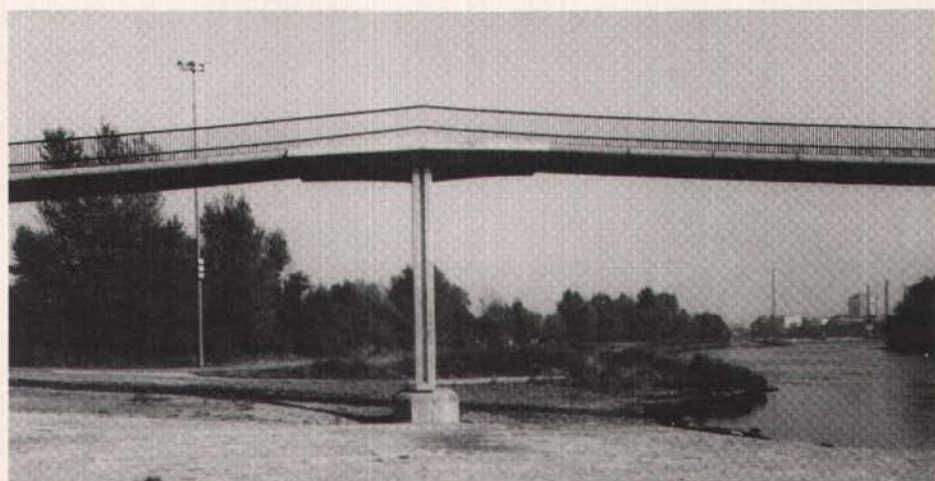
Fig. 11. Pedestrian bridge showing intermediate support.
