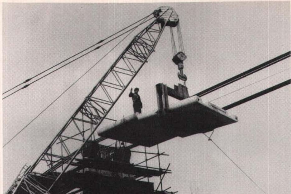
Fig. 15. Erection of a segment of the second span.
