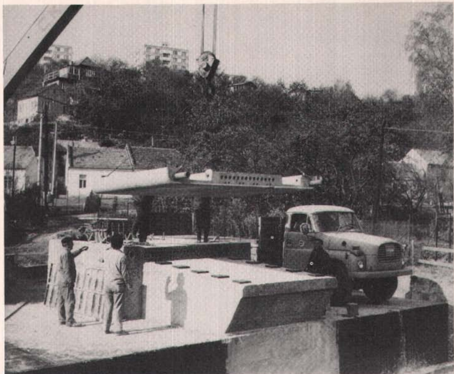
Fig. 13. Erection of the end segment.
