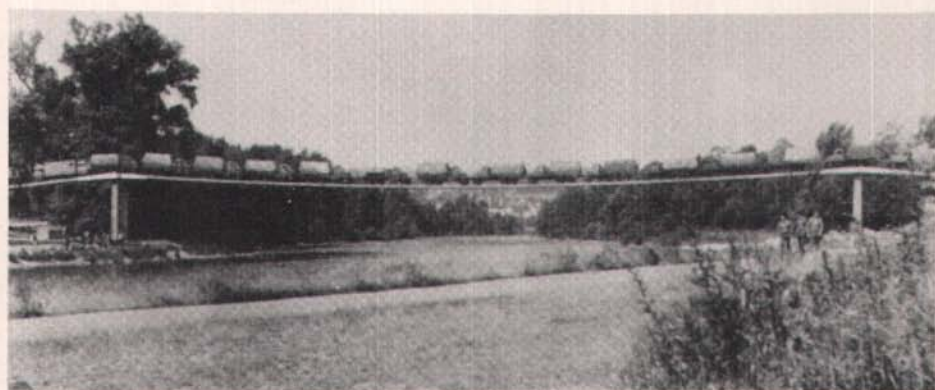
Fig. 20. Load test using 38 vehicles — Pedestrian bridge at Prague-Troja.
