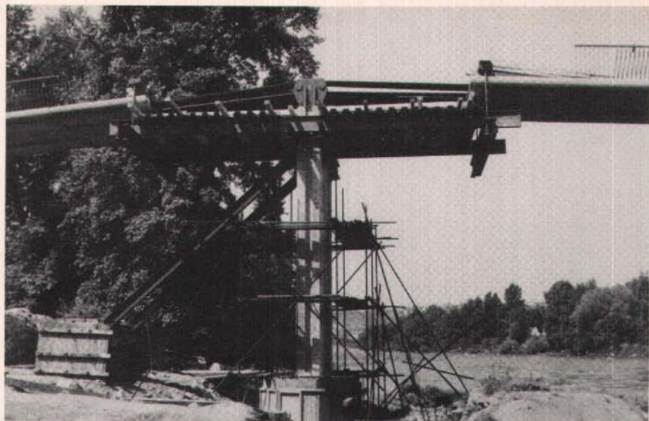
Fig. 17. Falsework of the saddle.
