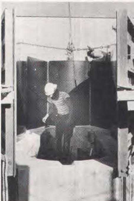
Fig. 6. The box piers were cast with a vertical match-cast system. Here the cast-against segment is being prepared for casting its neighbor on top.
