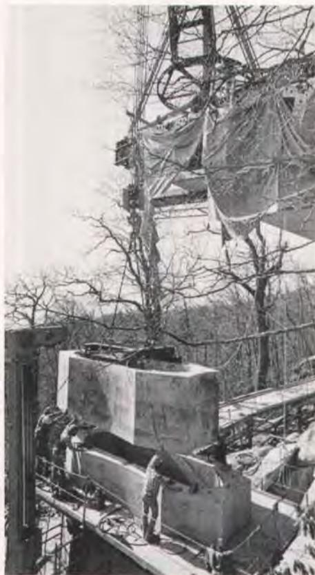
Fig. 9. Precast box pier segments were lowered over the end of the completed cantilever with the stiffleg. The workmen are ready to block the segment and apply the epoxy.
