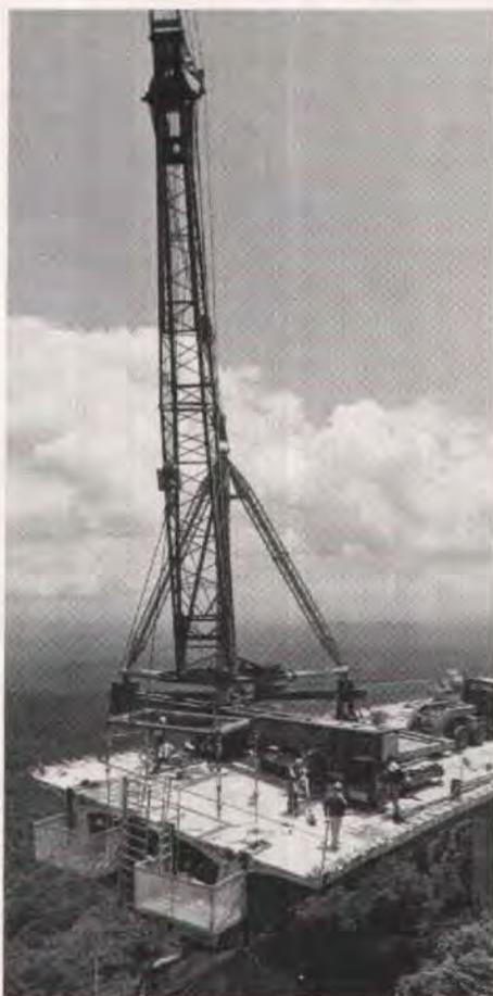
Fig. 8. The contractor chose to erect the segments with this stiffer crane attached to the end of the cantilever. This single piece of equipment controlled the construction rate of the bridge. All material and equipment was handled with this crane.
