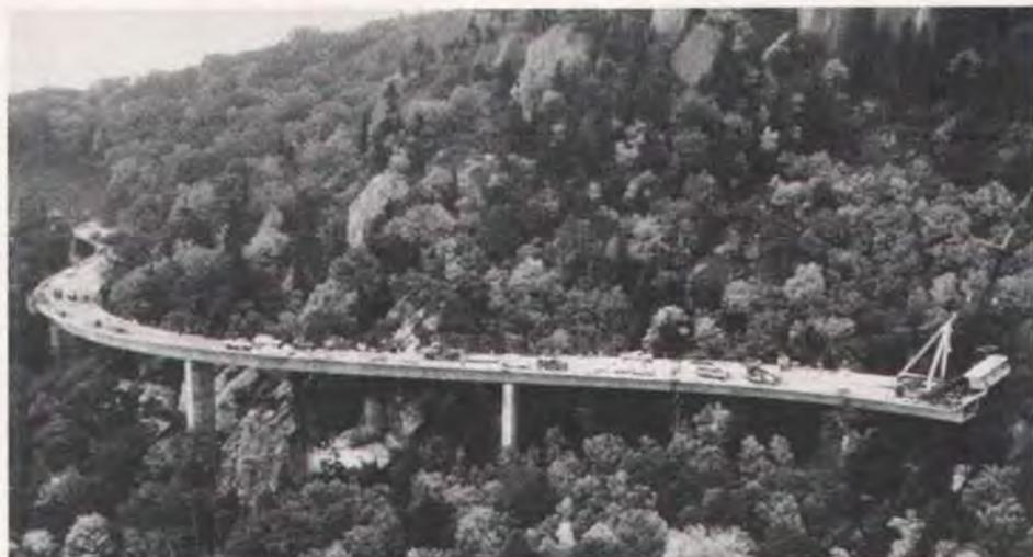
Fig. 2. Construction overview of Linn Cove Viaduct. This bridge is the first segmental structure in the United States to incorporate progressive placing erection.
