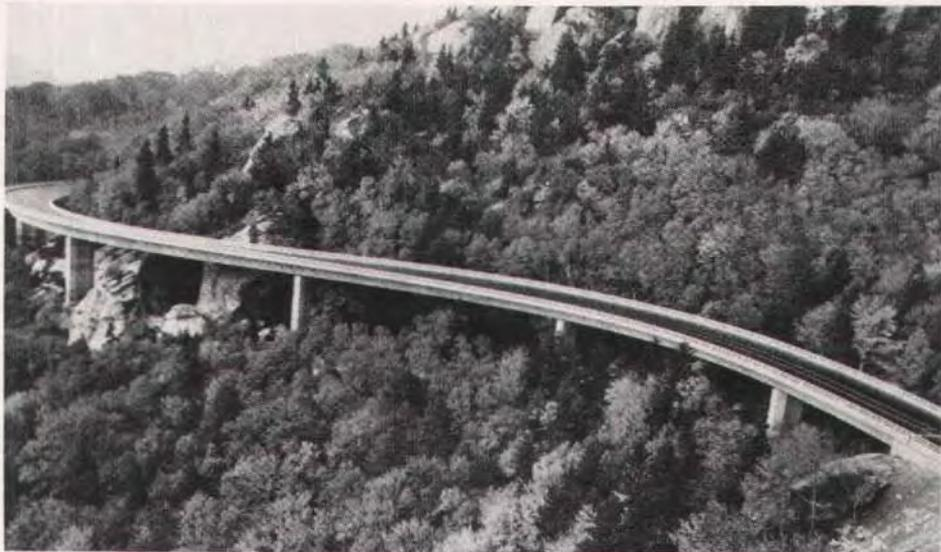
Several innovative design and construction techniques were used to build the Linn Cove Viaduct — a 1243 ft (379 m) long, S-shaped precast prestressed segmental concrete bridge — situated in one of the most scenically beautiful regions of the United States.
