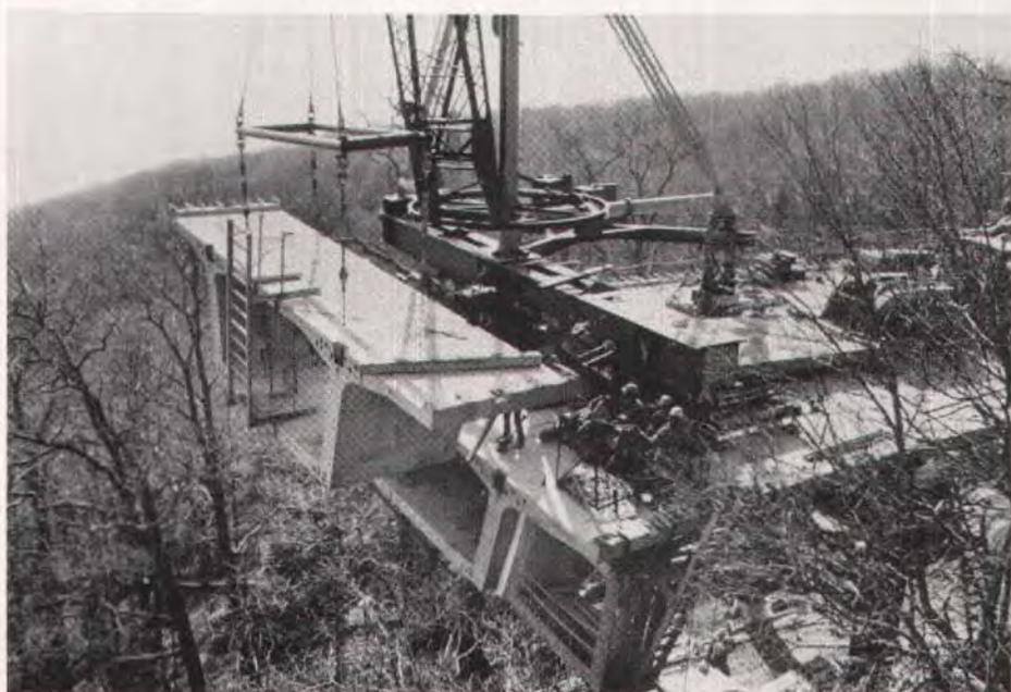
Fig. 13. Then the segment was lowered vertically.
