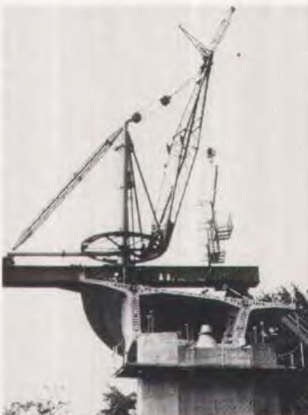
Fig. 11. The first step in the erection sequence was to remove the post-tensioning stressing cage from the end of the cantilever. The permanent tendon live end anchors can be seen at the top of the webs.
