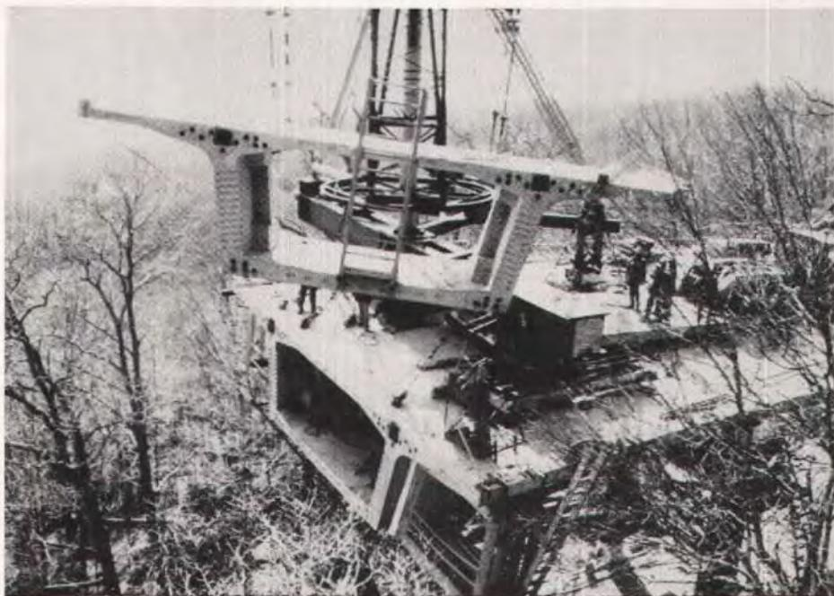
Fig. 12. The segment was lifted from the truck on the right and swung out over the cantilever end.
