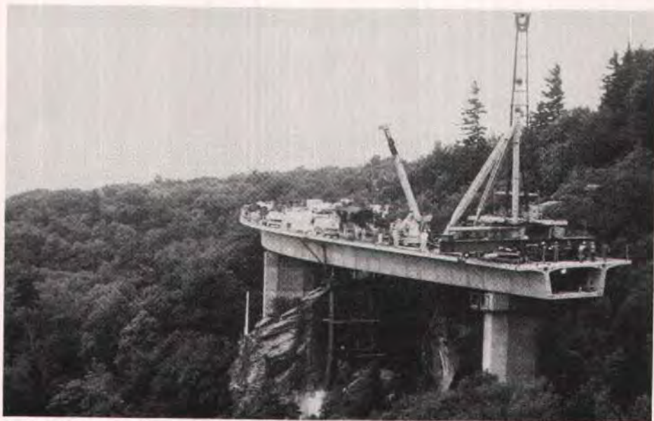
Fig. 8. Complex geometry at Linn Cove Bridge.
