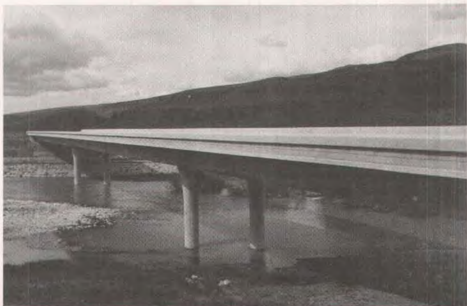
Fig. 13. Coyote Creek Bridge, Santa Clara County, California.
