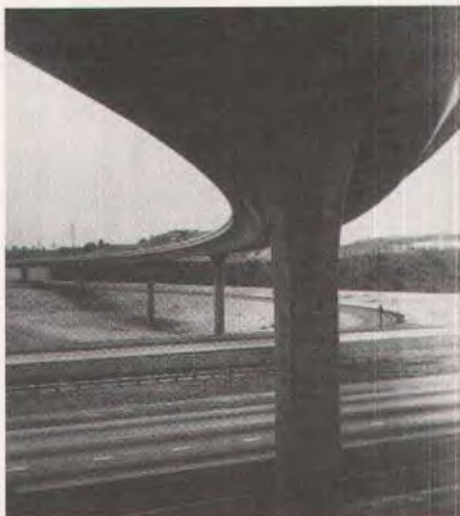
Fig. 12. Route 274/15 Interchange, San Diego County, California.
