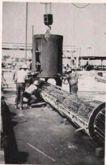
Fig. 23. Open form concrete placement (with reinforcement in place) used in manufacture of prestressed poles.
