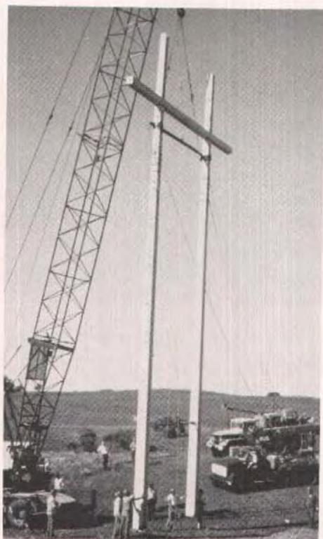
Fig. 38. Erection of an H-frame structure.
