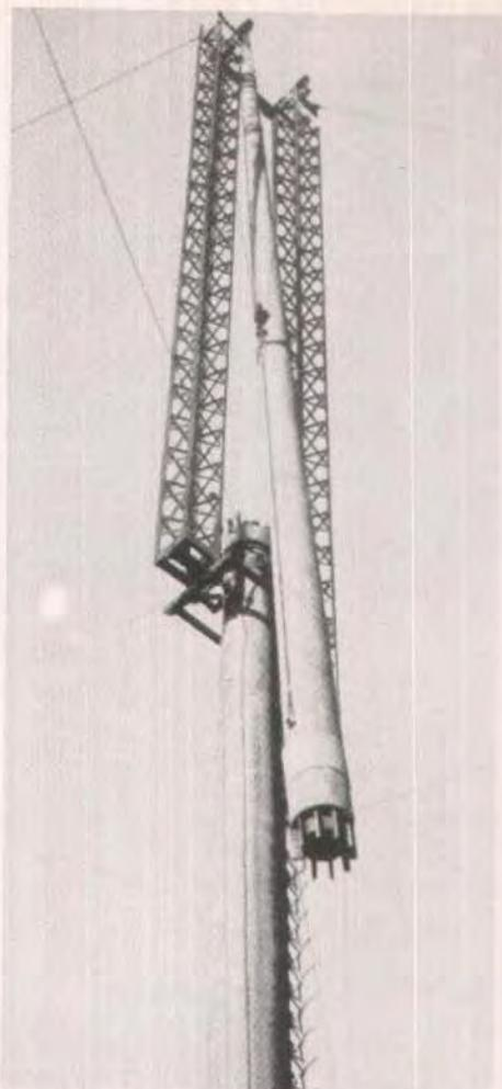
Fig. 37. Erection of a German two section bolted spliced structure.
