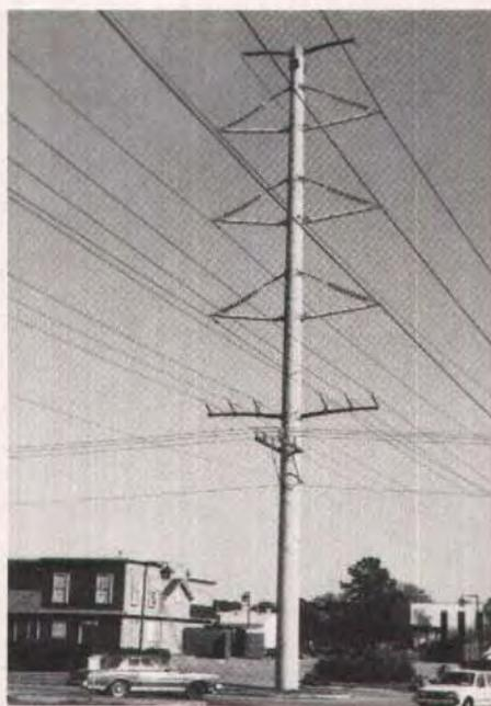
Fig. A13. Power transmission with distribution underbuild.
