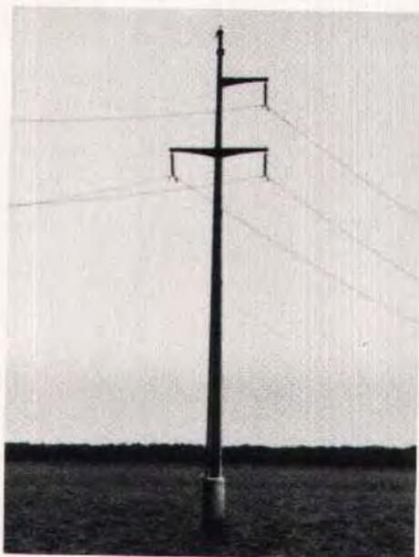
Fig. 17. Power transmission structure (Virginia Electric and Power Company Currituck Sound Crossing). Built in 1964, these tapered I-shaped prestressed concrete poles were used to upgrade a 34.5 to 11.5 kV, 3 mile (4.8 km) water crossing in North Carolina. The poles were manufactured using the centrifugally-spun cylinder pile method.
