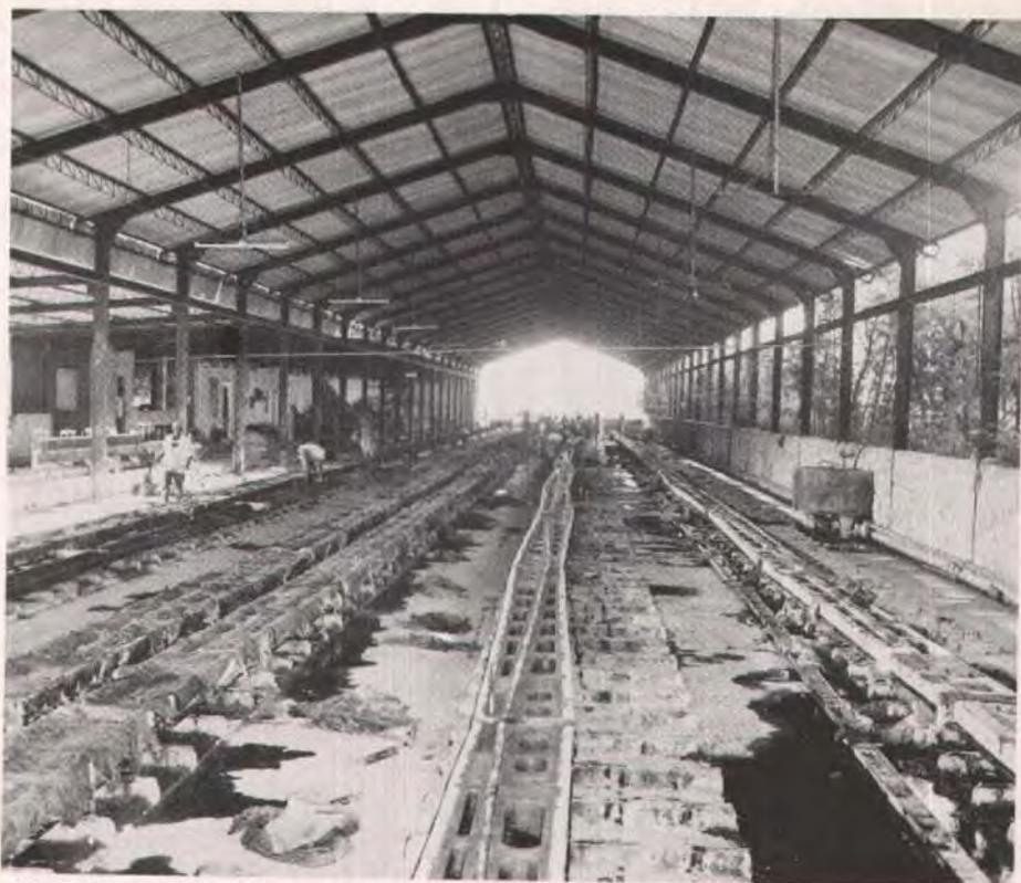
Fig. 27. Pole manufacture in India using Hoyer's long line method.
