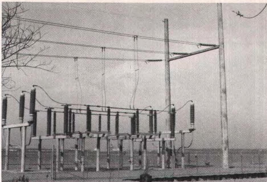
Fig. A27. Power overhead transmission to underground transmission.
