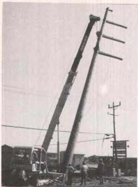
Fig. 36. Erection of a single pole structure.
