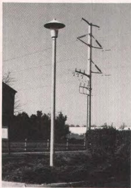
Fig. A12. Power transmission with distribution underbuild and area lighting.
