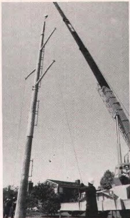
Fig. 41a. Slip joint splice.
