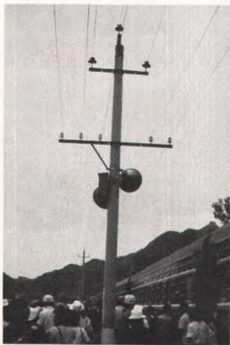
Fig. 2. Closeup of spun concrete pole (Shanghai Electricity Bureau).
