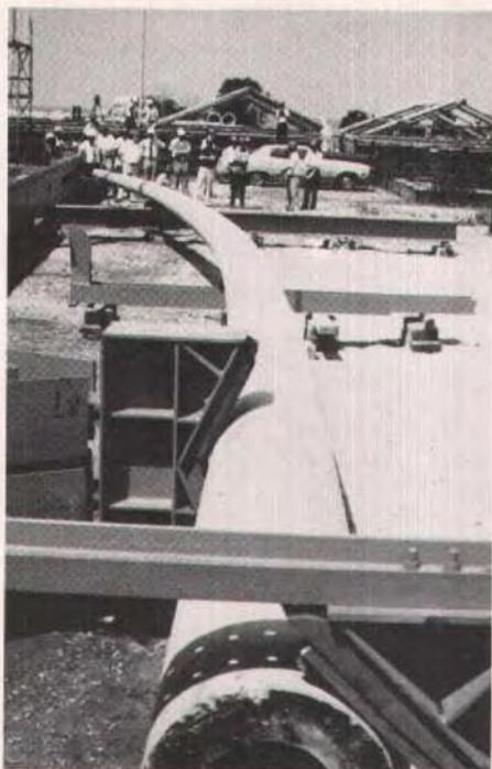
Fig. 28. Horizontal testing of concrete pole for flexural capacity.
