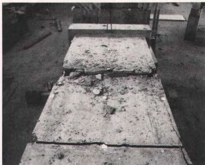
Fig. 29. Specimen 1 — Top plate — View of top plate looking west showing buckling of west plate over east plate. Diagram at right shows orientation of specimen and location of failure.
