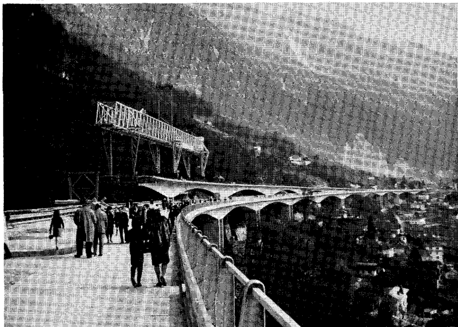
Fig. 20. Chillon Viaduct, Switzerland.
