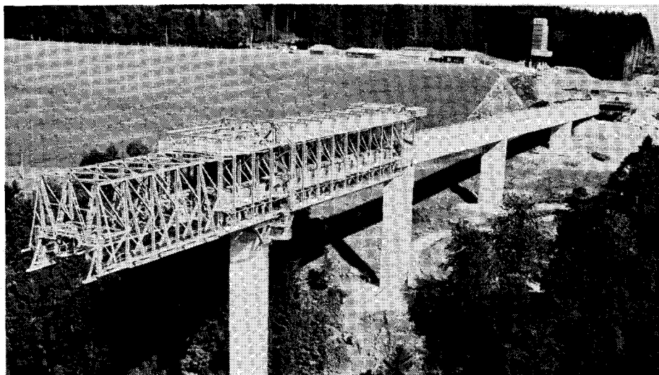
Fig. 7. Gruyère Viaduct, Switzerland. Launching truss in operation.
