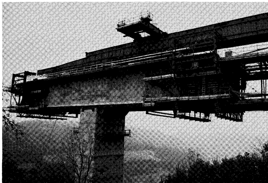
Fig. 15. Kochertal Bridge, Federal Republic of Germany. Launching girder and travellers.
