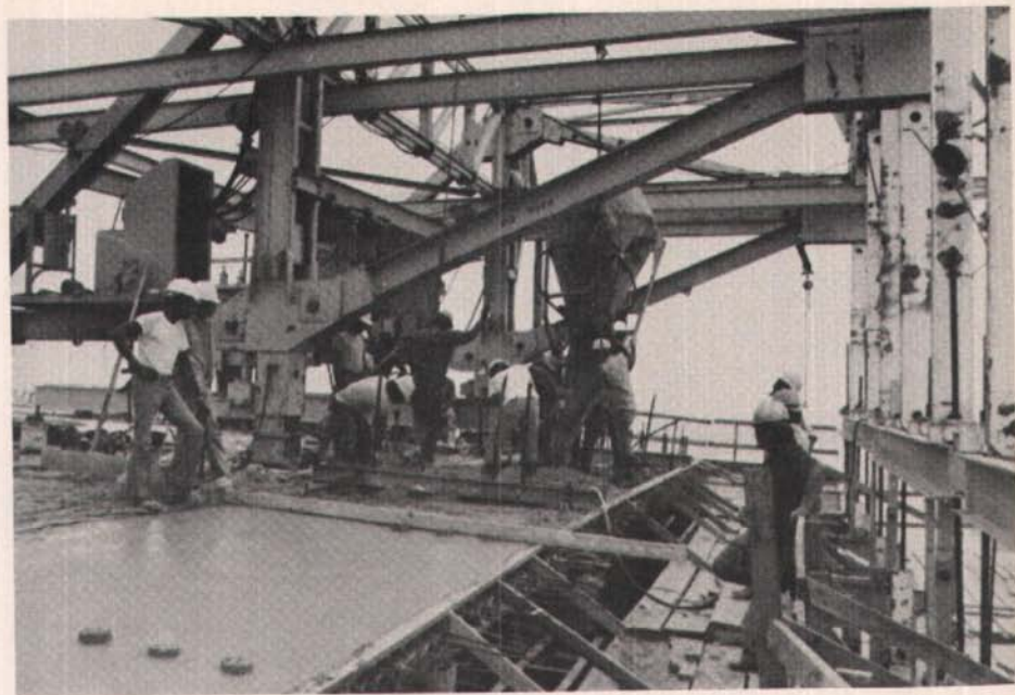
Fig. 16. Concrete placement with crane and bucket.
