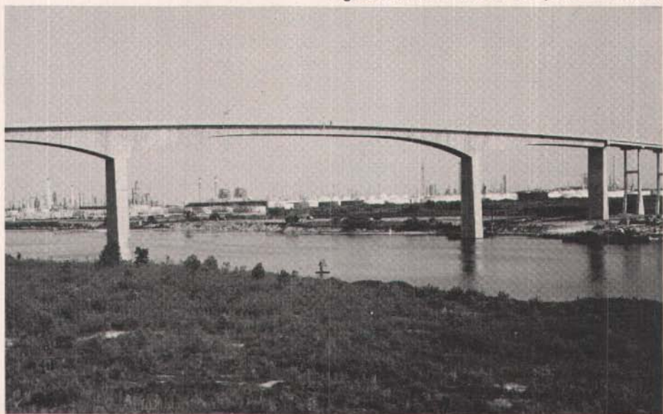
Fig. 23. Another view of completed structure.
