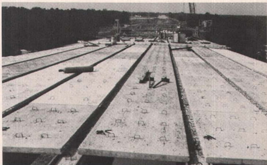
Fig. 9. Precast prestressed concrete deck panels used on land approaches.
