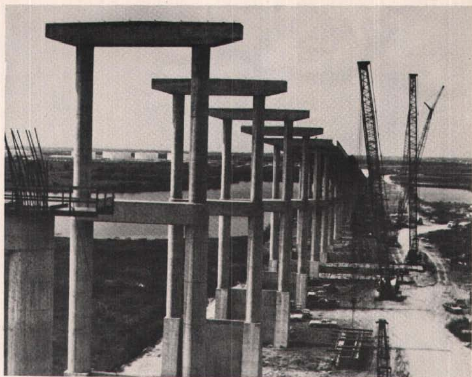
Fig. 7. Piers on land approaches.
