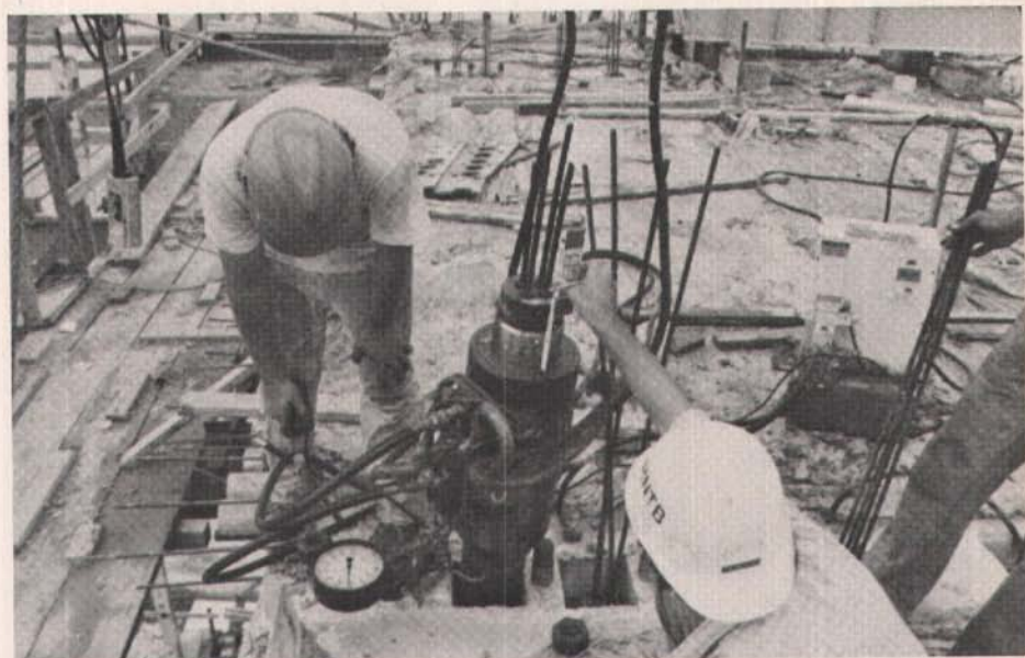
Fig. 18. Stressing of vertical tendons.
