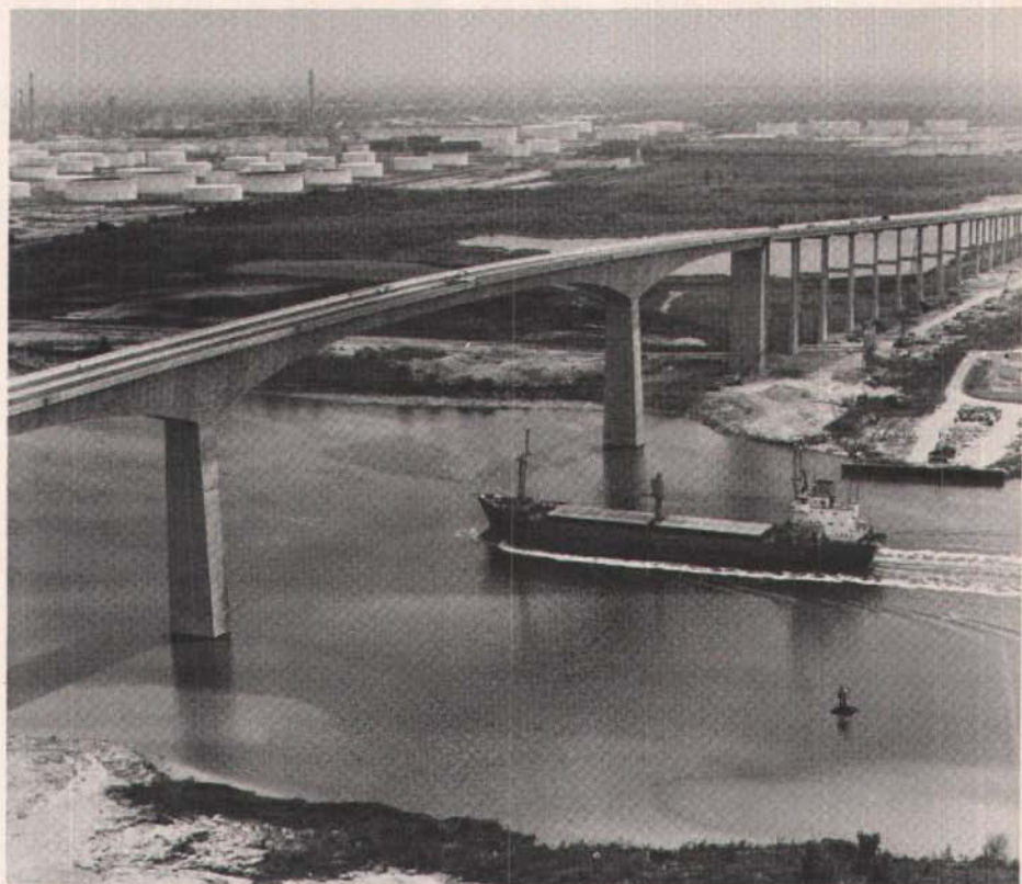
Fig. 22. Houston Ship Channel Bridge in use.
