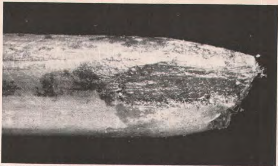
Fig. 8. Surface of wire sample adjacent to fracture showing elongated corrosion pits which intersect the fracture.
