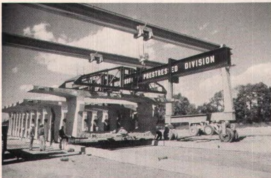
Fig. 15. Once the length of the bed was produced the segments were stored in the yard to await delivery.
