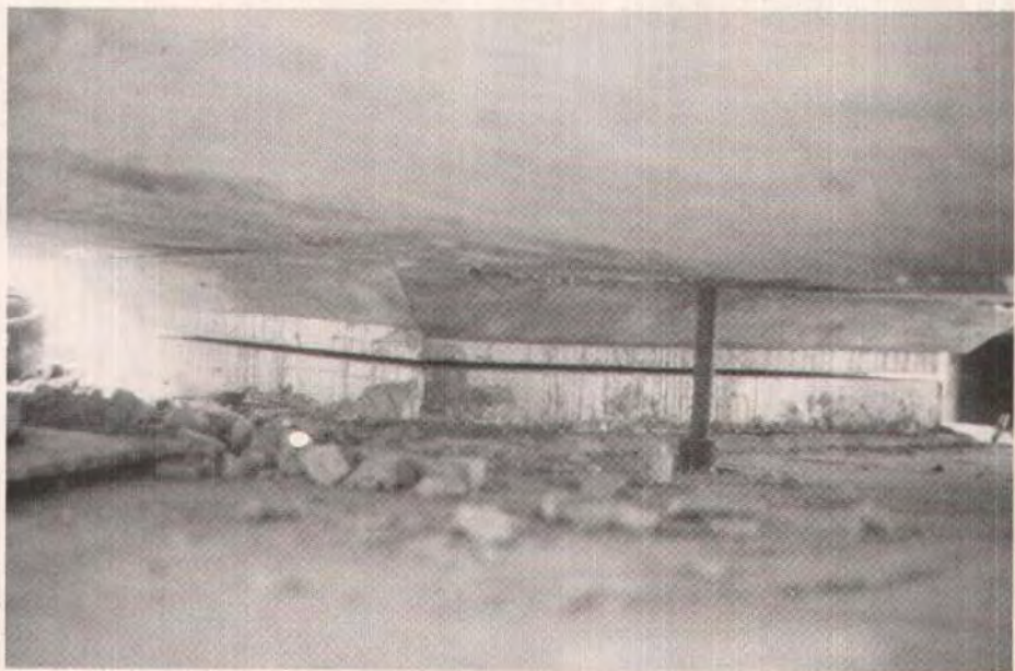
Fig. 24. The pot bearings were grouted in place after the balanced cantilevers were lined up.
