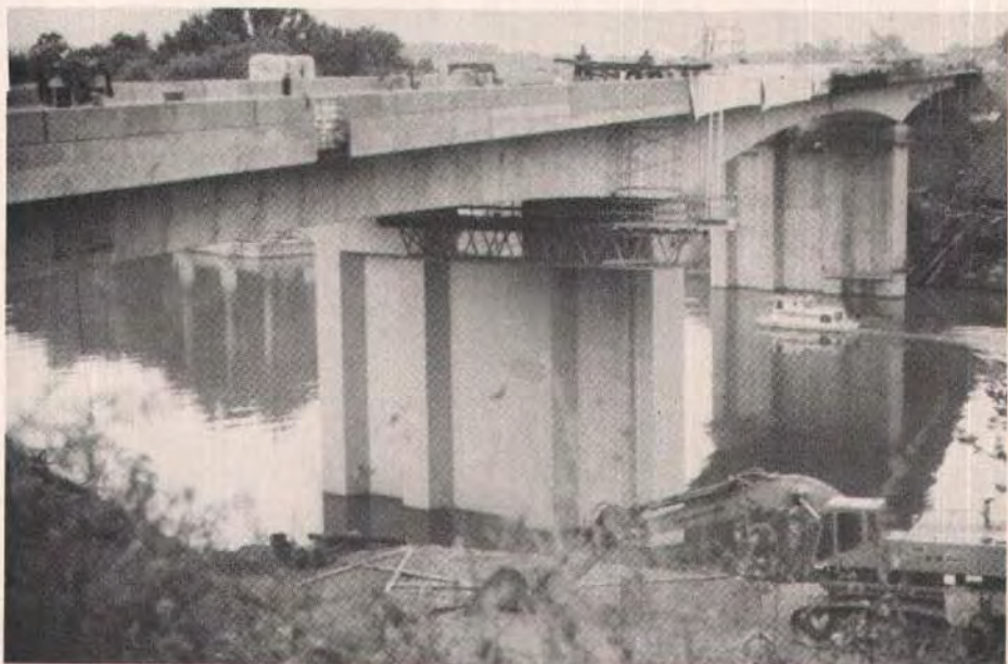
Fig. 28. The final cleanup just prior to final completion of the structure.
