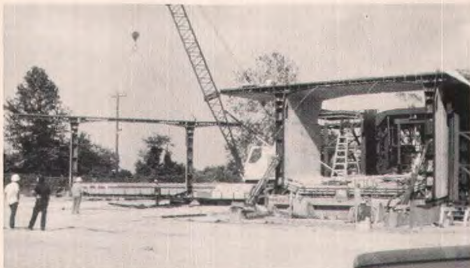
Fig. 9. First segments produced showing view of adjustable bulkhead.
