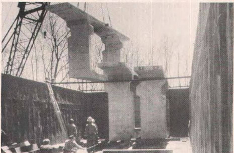
Fig. 17. The deeper segments were loaded on barges.
