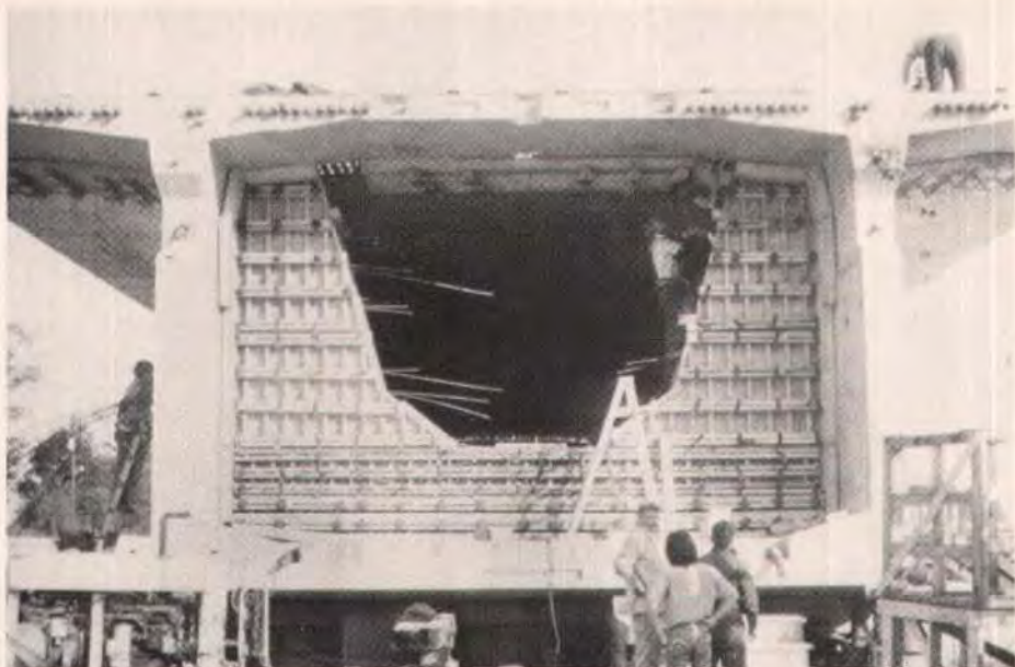
Fig. 13. The heavy pier diaphragm was also formed with wood.
