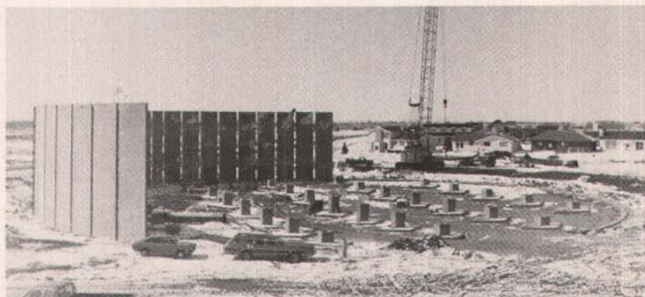
Erection of wall panels in late winter showing column pedestals and perimeter footing (March 1979).
