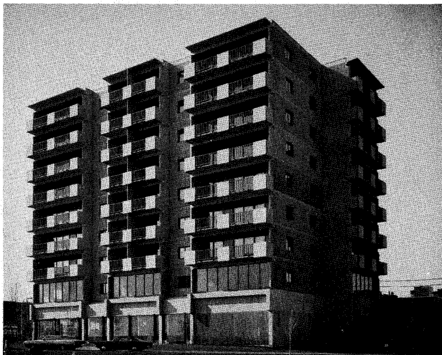
Fig. 1. Geneva Towers, Lake Geneva, Wisconsin. This nine-story condominium and office building used 245 6-in. (152 mm) thick loadbearing wall panels with sizes up to 10 ft high x 42 ft long (3.05 x 12.81 m). Double-tees were used for the floor and roof members.
