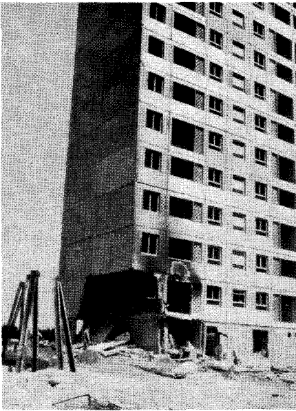
Fig. 8. Algerian bearing wall concrete building which survived a major explosion (Reference 1).
