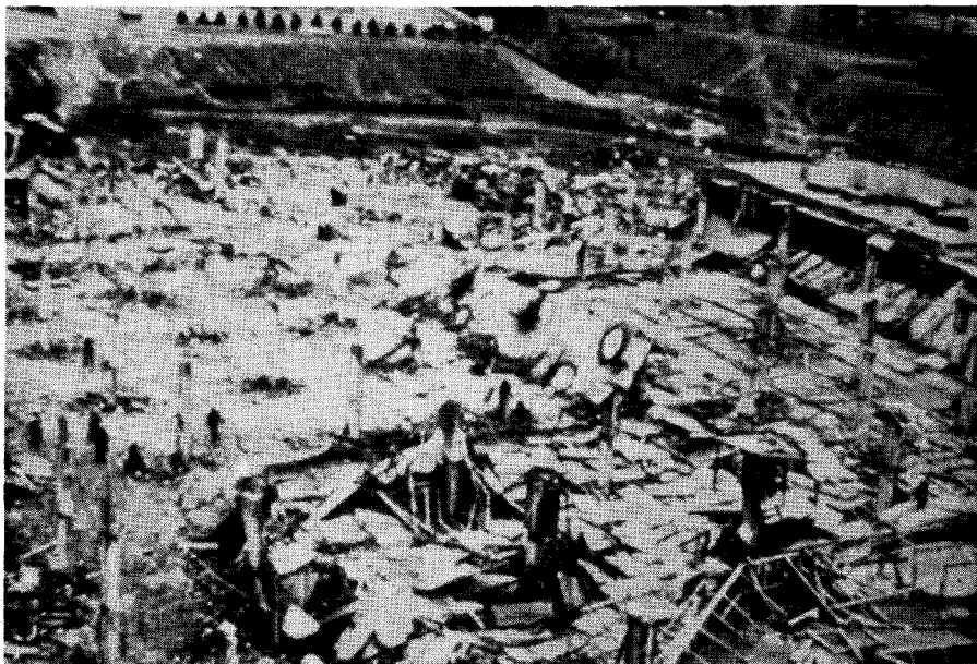
Fig. 7. Collapse of cast-in-place post-tensioned parking garage which was struck at one edge by falling tower crane and debris (Bailey's Crossroads, Virginia).
