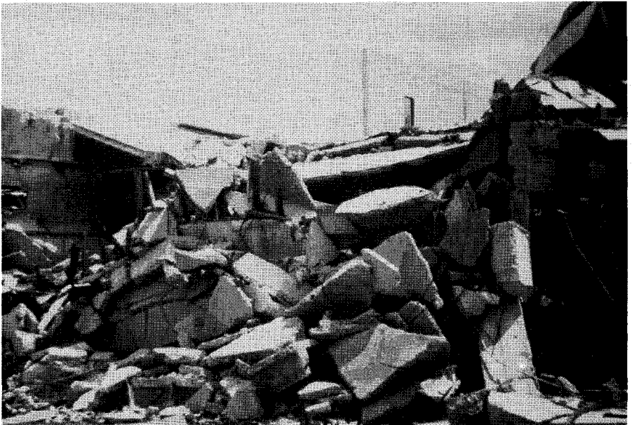
Fig. 16. Two-story tiltup bearing wall building with grossly inadequate connection details (Baton Rouge, Louisiana).
