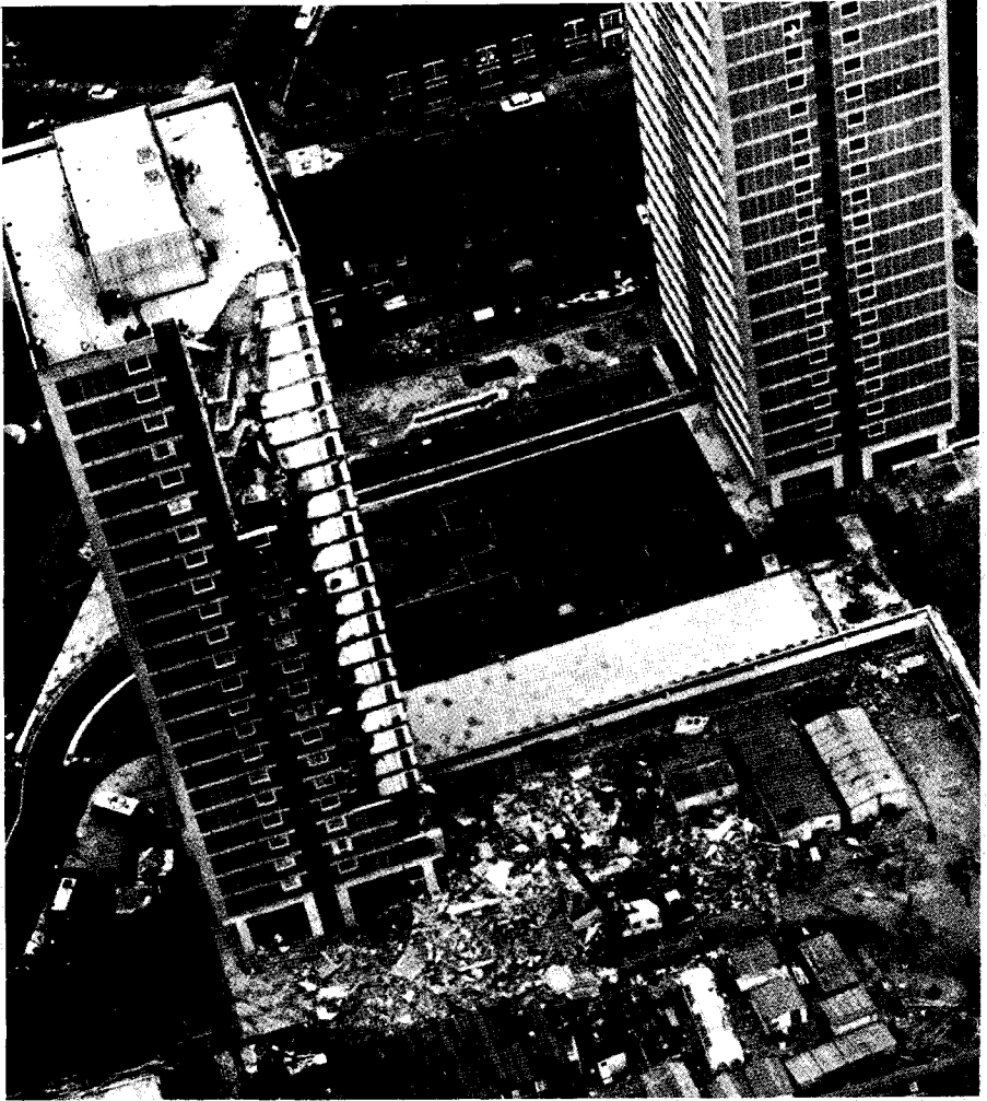
Fig. 5a. Ronan Point Apartment Building after collapse, with a second identical building in background. (Courtesy: London Express News and Feature Services.)
