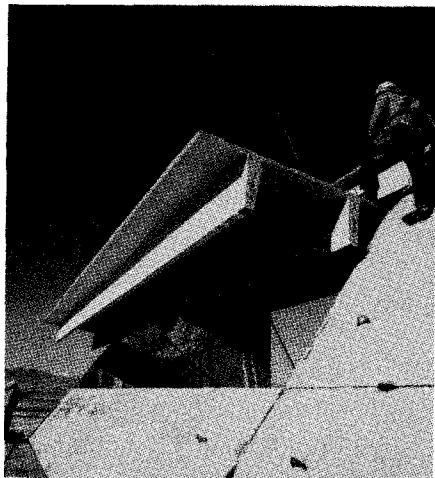
Precast double tee being moved prior to tilting on roof.
