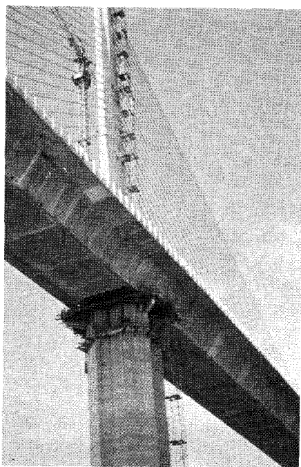
Fig. 29. Bottom view of deck segments of Pont de Brotonne near Rouen, France.
