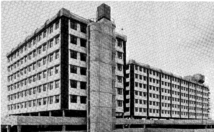
Fig. 13. Double skin window and mullion panels on office block development at Kingston on Thames, England.
