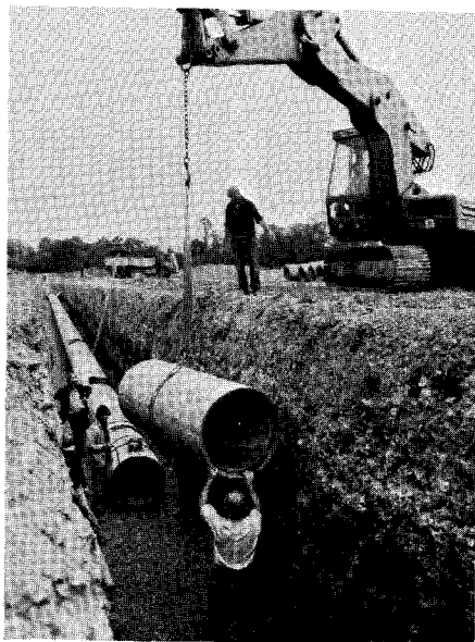
Fig. 5. 30-in. diameter GRC concrete pipes manufactured in England using centrifugal spinning process.
