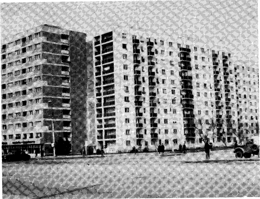
Precast buildings designed to withstand quakes held up well.
