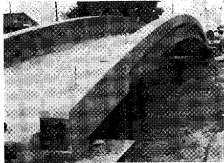
Fig. 5b. Completed span after stressing.
