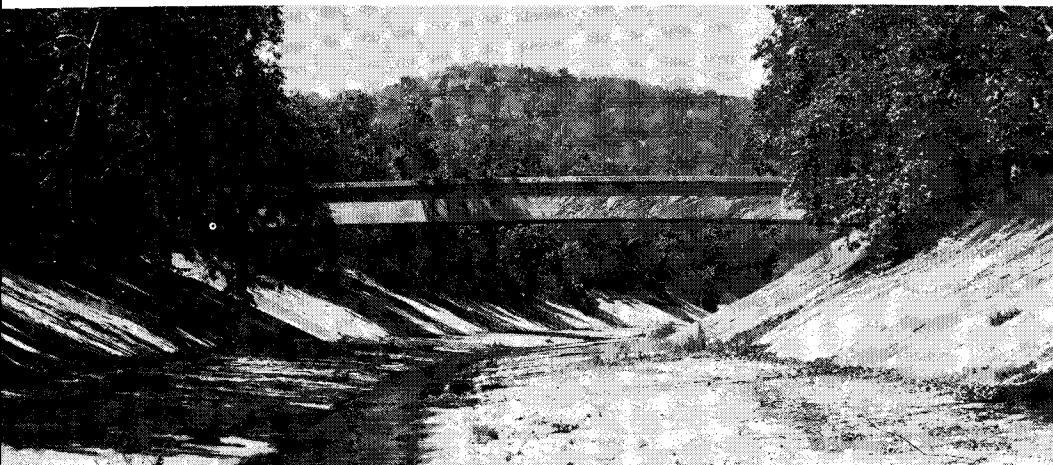
Fig. 1. Arroyo Seco Pedestrian Overcrossing.
