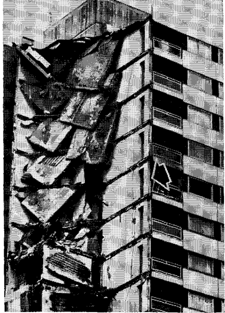
Fig. 3. Collapse at Ronan Point.
