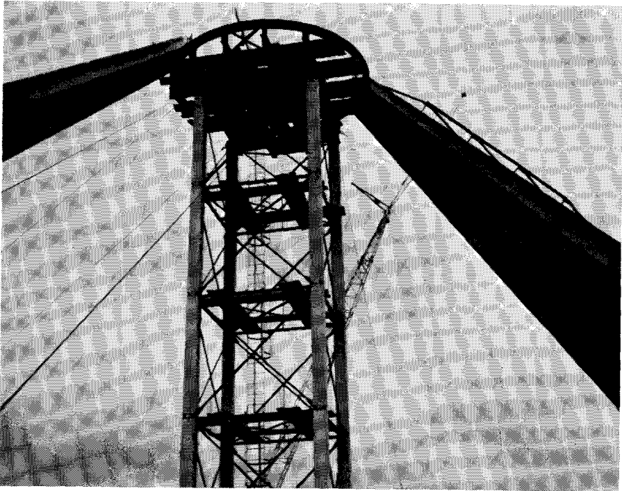
Fig. 18. Close-up of temporary erection tower.
