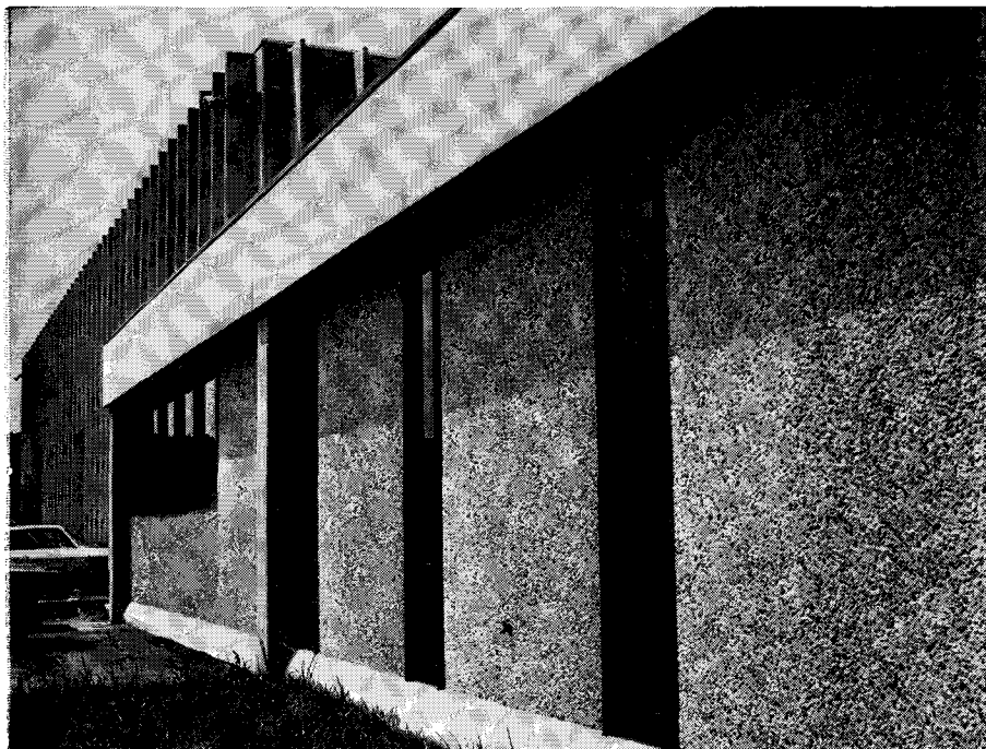
Closeup of office building showing exposed aggregate precast wall panels.
