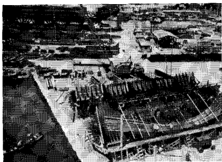
Fig. 7. Fabrication of anchorage beam
