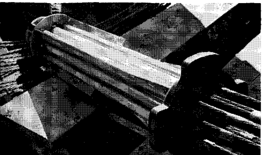
Fig. 16. The aluminum alignment cartridge is placed on the tendon prior to attaching the jacking ram.
