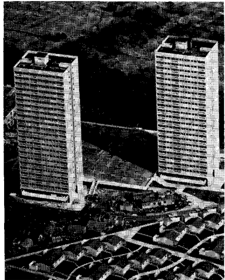
Fig. 3. Multi-storey Bison Wall Frame apartment blocks, Leicester, England
