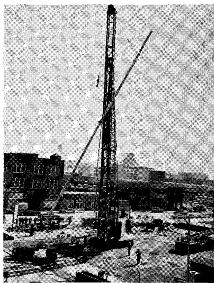
Fig. 2. Long foundation pile (without splices) being used for construction in an American city
