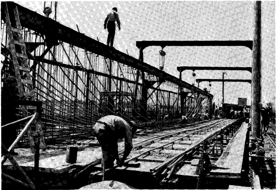
Fig. 3—Preparation of a Cable and Reinforcement Cage for T-Girders
