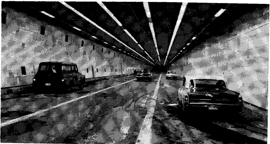
Fig. 7—Interior of Completed Lafontaine Tunnel
