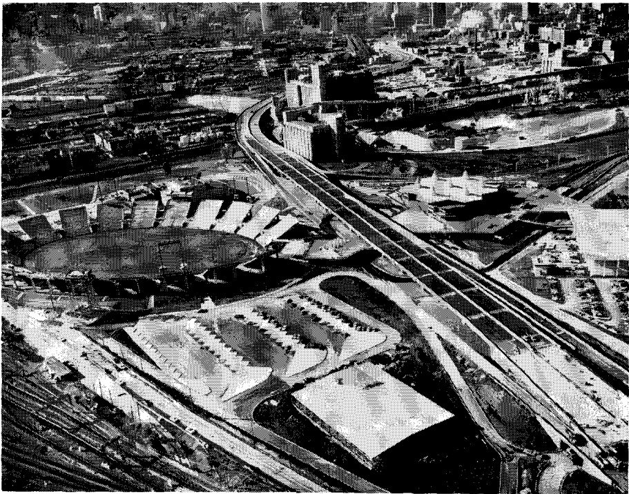
Fig. 9—Bonaventure Autoroute Skirts Expo 67, Montreal
