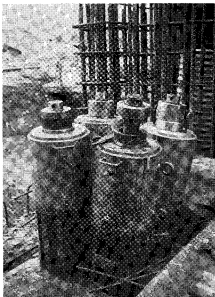
Fig. 16—Four 500-Ton Jacks for Stressing an Anchor
