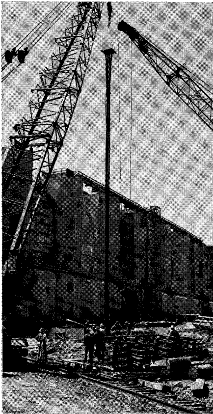
Fig. 14—Crane Lifting an Anchor
