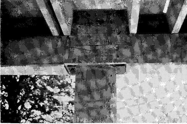
Fig. 7—Horizontal plate haunch BC(a).
