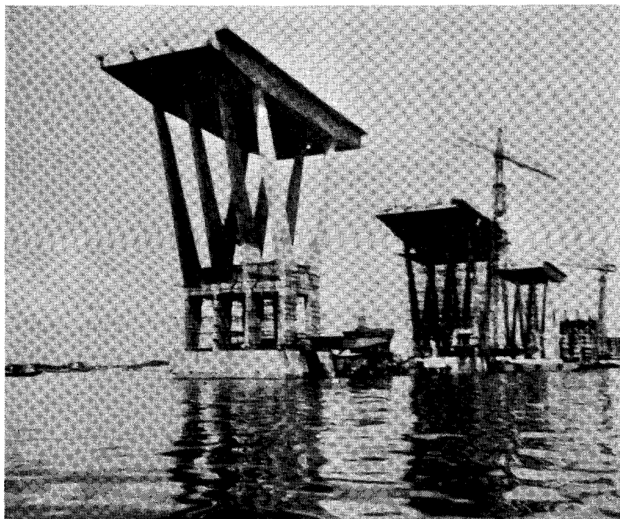
Fig. 16—Pier and Beam Construction 279 ft. Span
