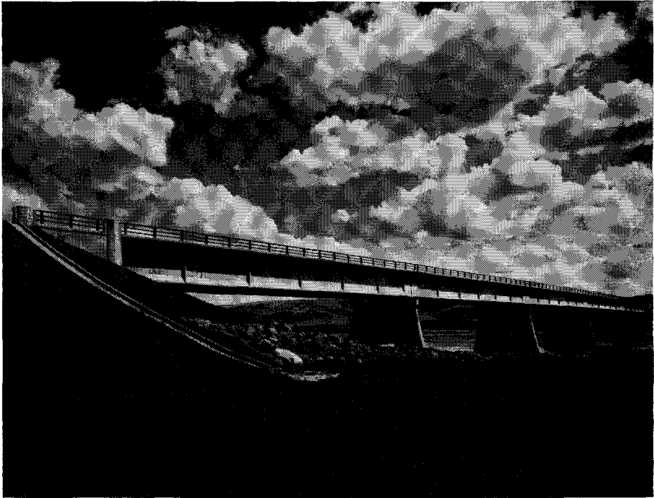
Fig. 10—Graceful lines of completed structure are emphasized in this photo.
